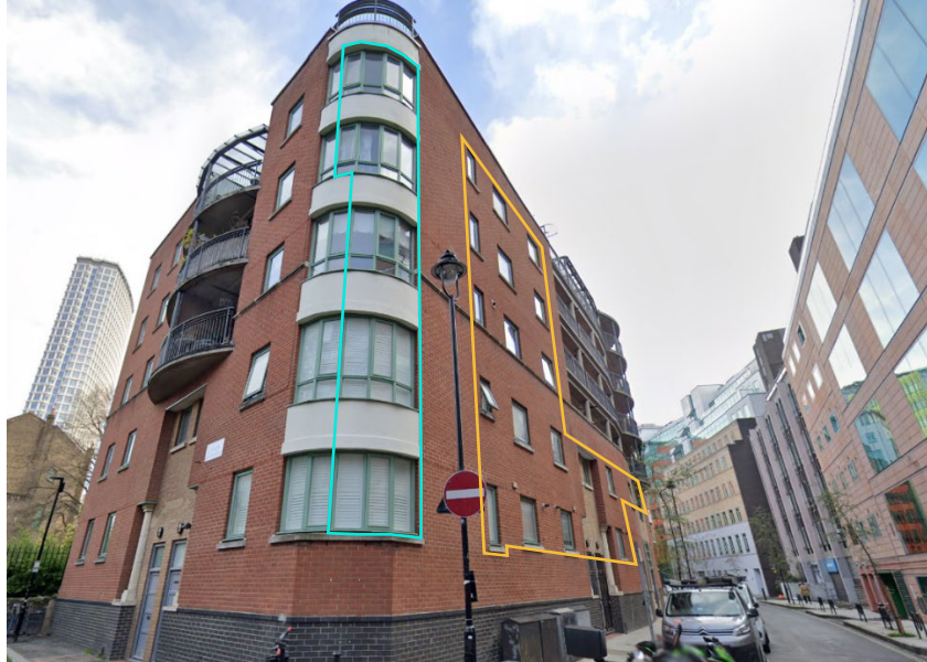
Figure 8 – Pendrell House. Windows with potential VSC impacts beyond BRE guidelines are outlined in colour: cyan = Saville Theatre, yellow = 151 Shaftesbury Avenue
