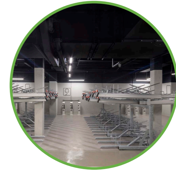
TRANSPORT HUB BY PROVIDING A FULLY EQUIPPED CYCLE STORE WE'LL BE PROMOTING MORE SUSTAINABLE MODES OF TRANSPORT AND PHYSICAL ACTIVITY.
