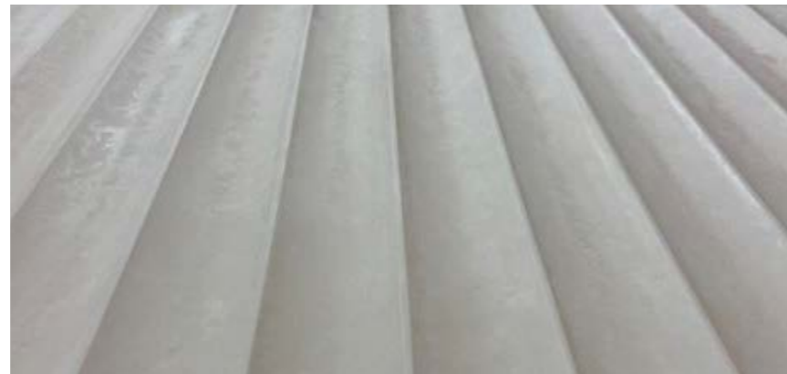
GRC PANELS TO UPPER FLOORS, CORNER AND LINTELS
