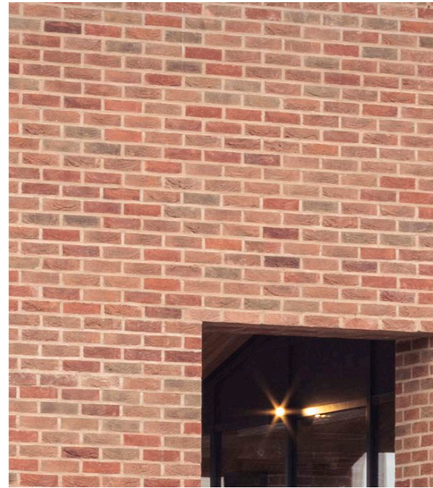
PANELISED BRICK FACADE / RECYCLED CONTENT
