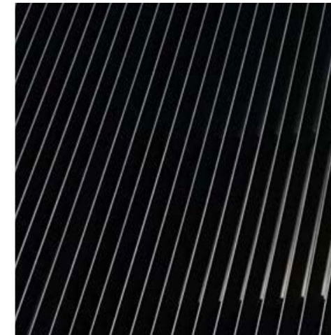
PPC METAL LOUVRES ABOVE WINDOWS AND OPENABLE SIDE VENTS
