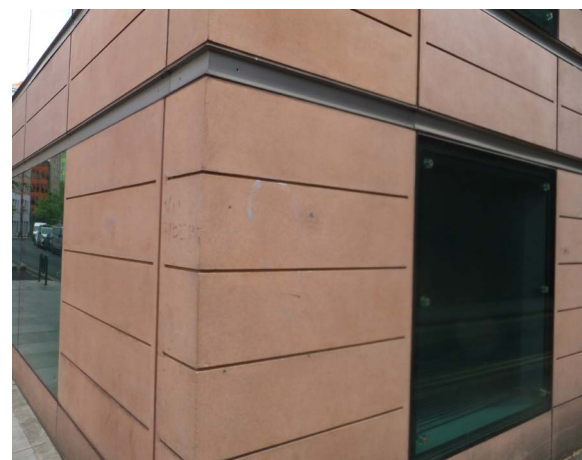
⑥ SHAFTESBURY AVENUE FACADE AND CORNER TO ST GILES PASSAGE
