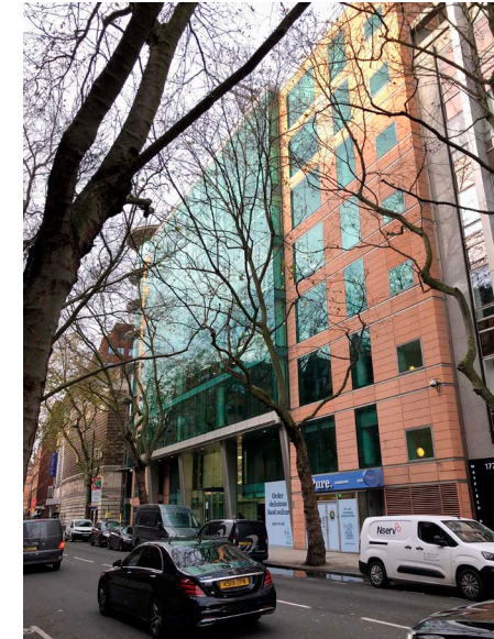
② 151 SHAFTESBURY AVENUE FACADE
