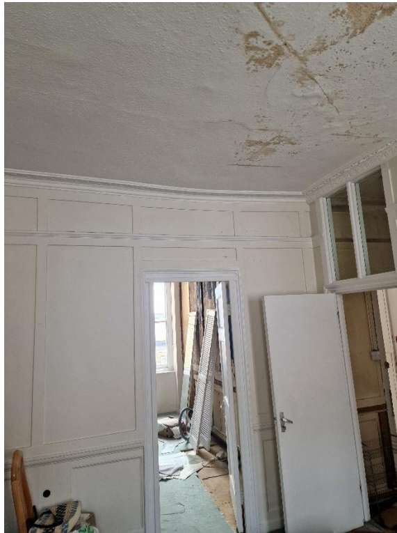
Figure 4 - Vertical movement in the ceiling/floor at 45 Great Ormond Street
