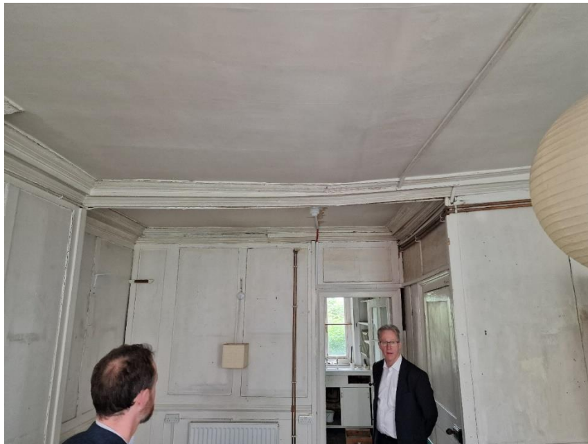
Figure 5 - Vertical movement in the ceiling/floor at 51 Great Ormond Street
