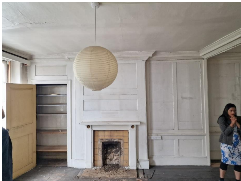
Figure 4 - Vertical movement in the ceiling/floor at 51 Great Ormond Street
