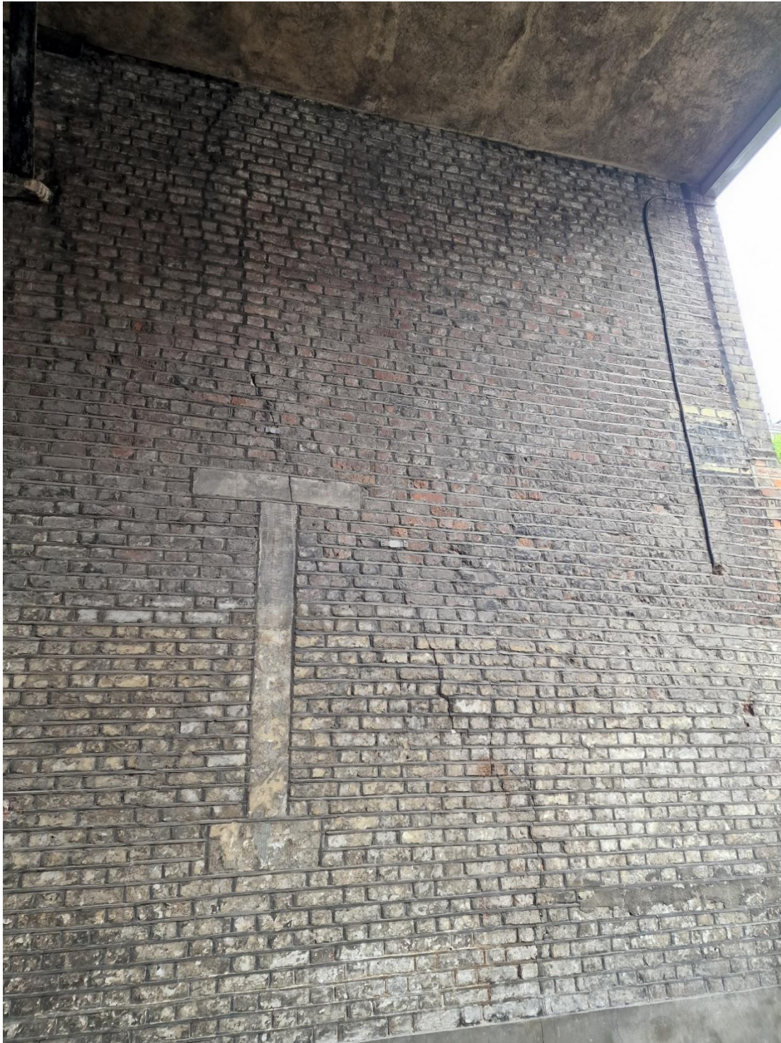
Figure 6 - Crack in External wall at Barbon Close
