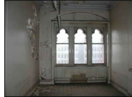
4 - South elevation of 3.098 with paint flaking
