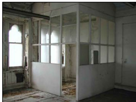
8 - South wall of 3.097 with deteriorating panelling under window
