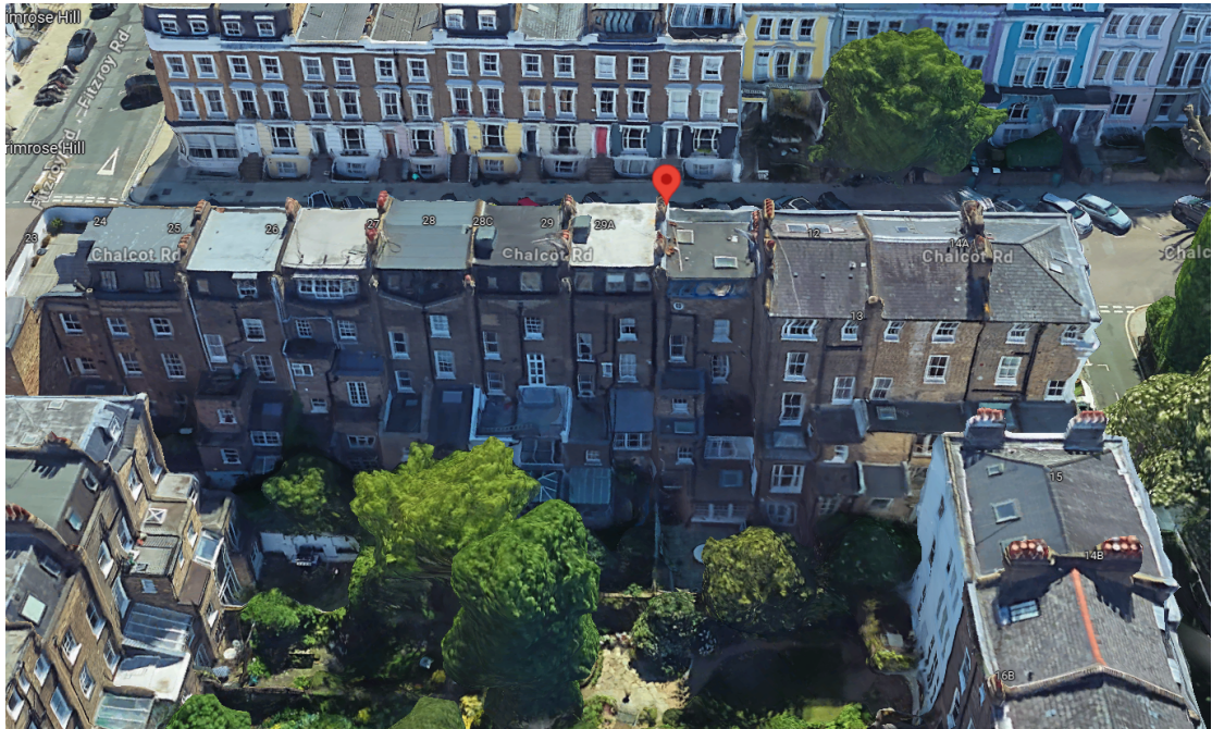
Aerial view of rear of 30 Chalcot Road and the terrace.
