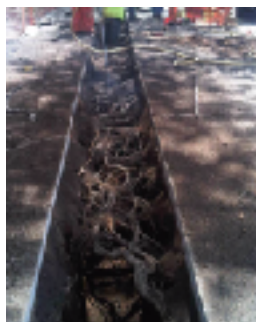
Example imagery of air spade use for implementing utilities beneath root plate (existing)
