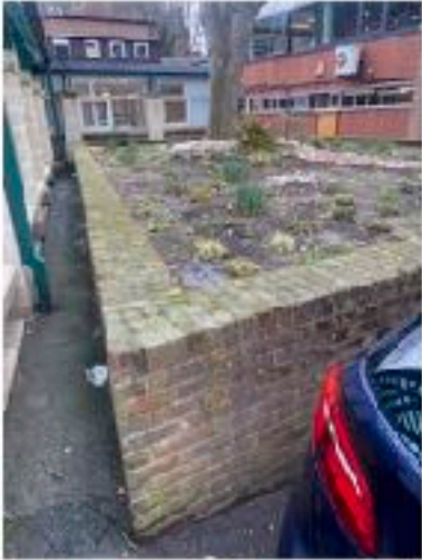
Tree T1 viewed to south showing raised retainer
