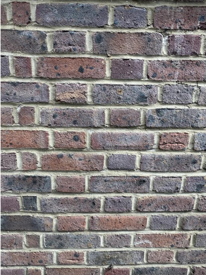
1. Existing Brick Work
