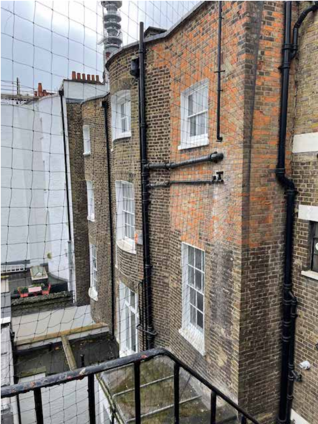
PHOTO F – Rear façade of residential properties in Fitzroy Street
