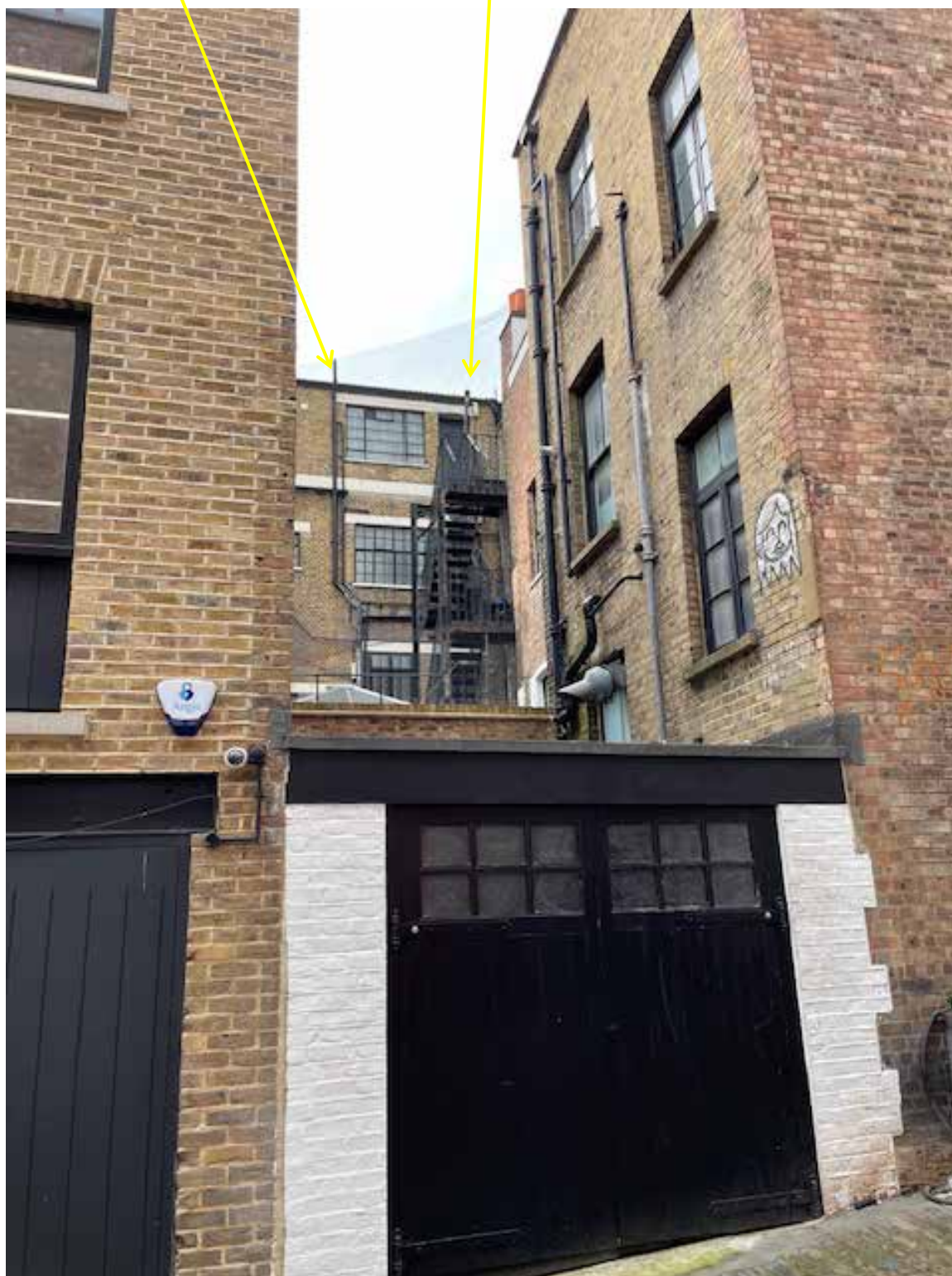
PHOTO D – Rear view of 22 Warren Street from Grafton Mews with microphone B at top of fire escape stairs
