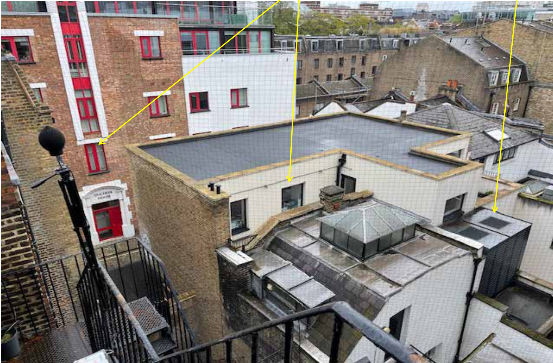
PHOTO E – Microphone B at top of fire escape staircase at rear of the building
