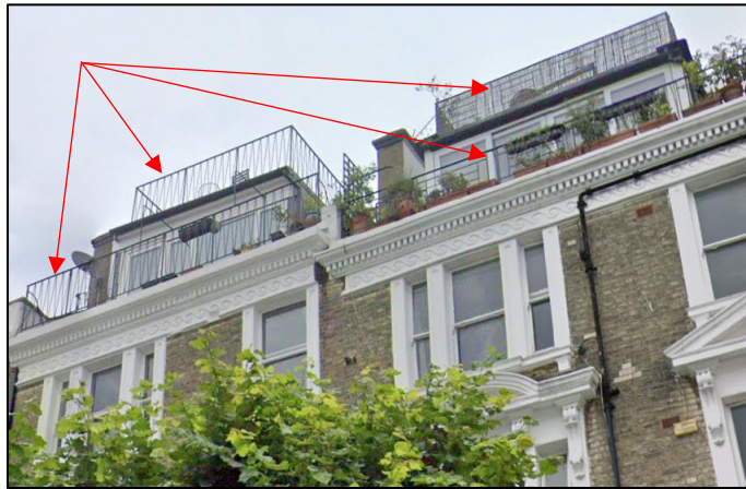
Metal balustrades to roof terraces
