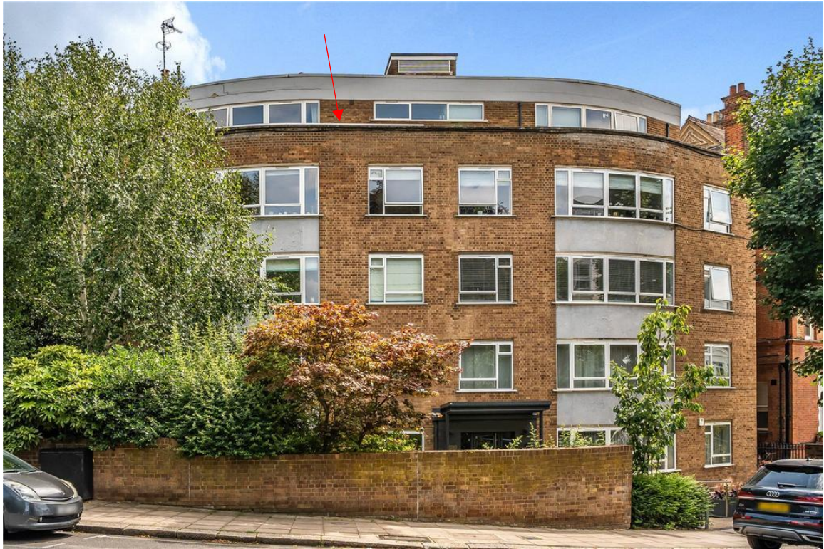
Figure 3 – Akenside Court, front elevation; relevant area shown by arrow
