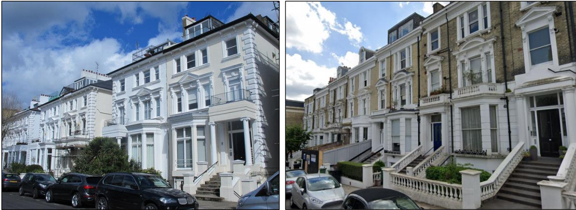
Figure 9 –Victorian Housing along Belsize Park Gardens and right, Belsize Crescent
