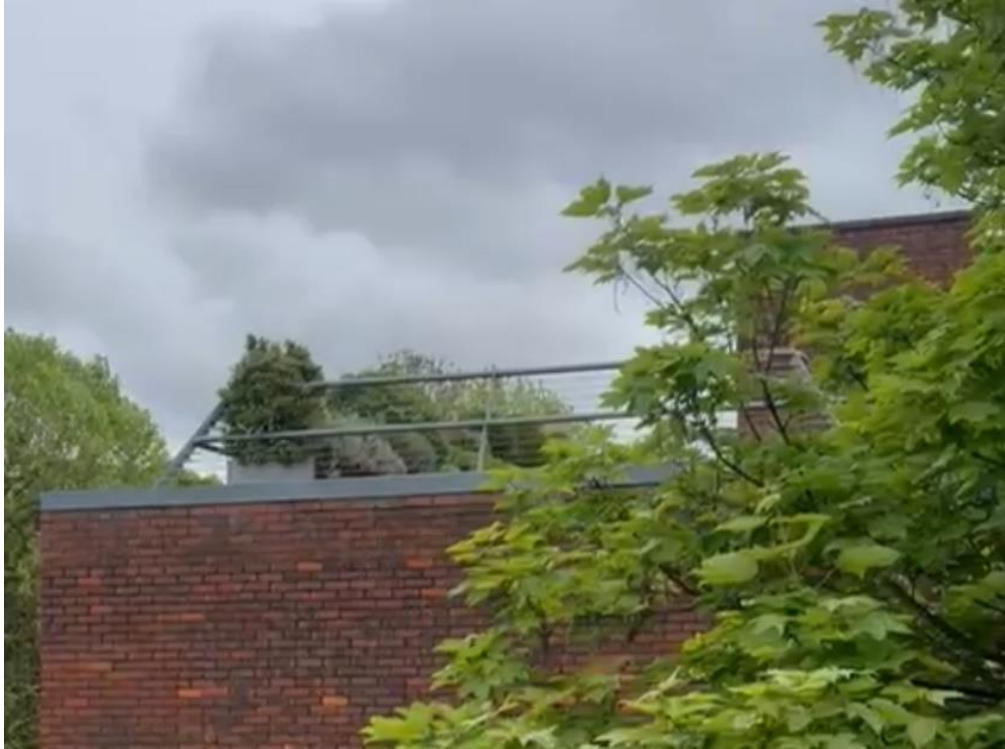
Figure 27– Neighbouring the site – a much more visually dominant metal balustrade to the rooftop of Roscommon House
