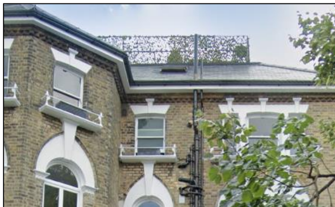
Metal balustrades to roof terraces
