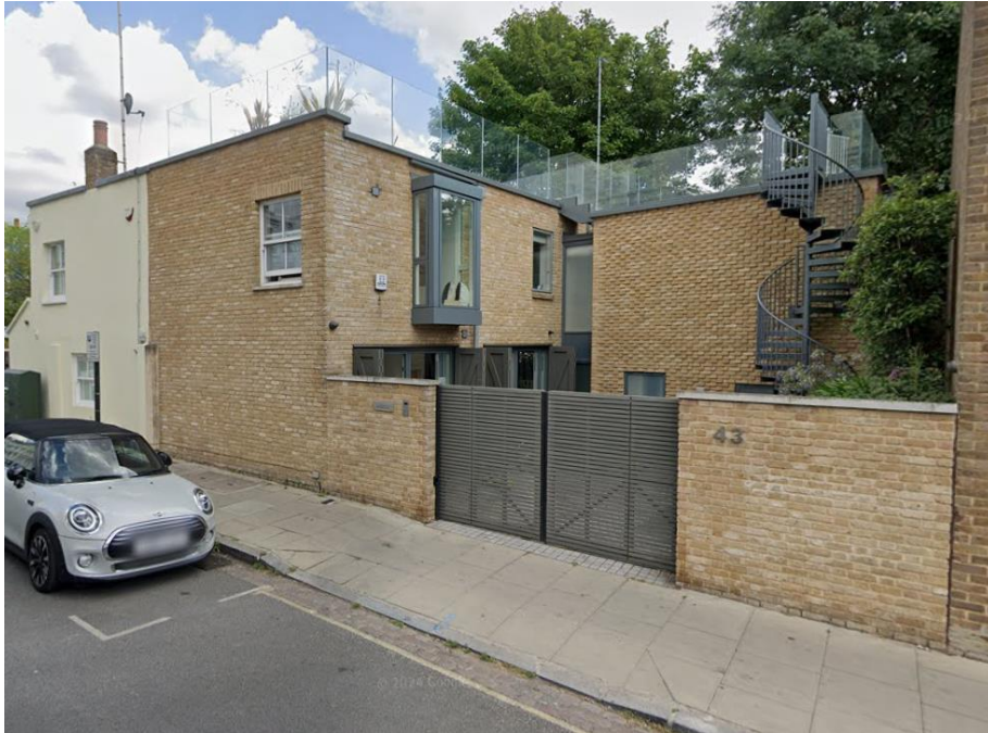
Figure 25 - glass balustrade at 43 Belsize Lane
