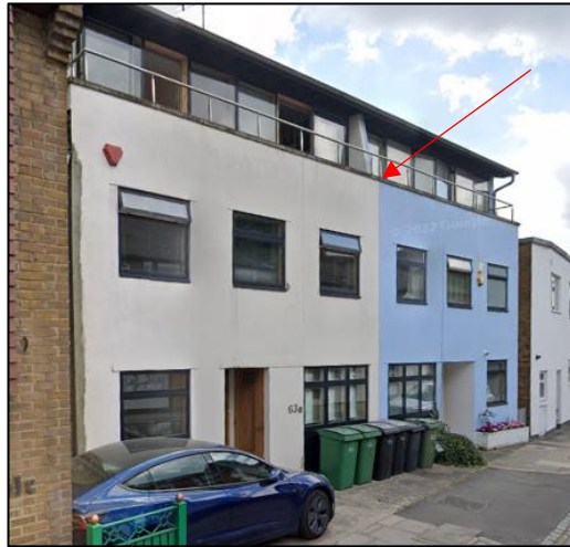
Metal balustrade to roof terrace
