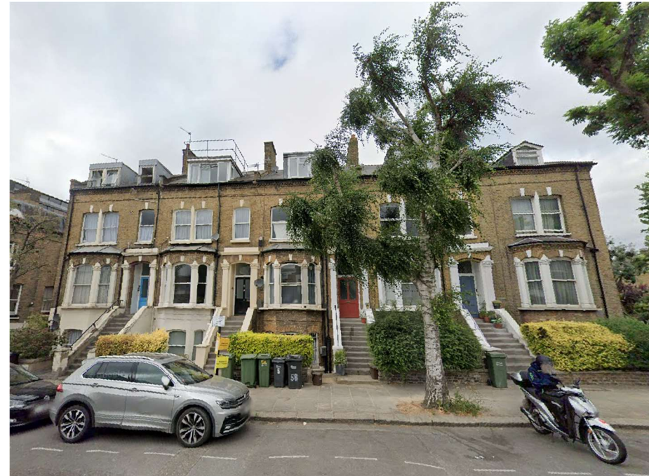
Fig 2 / Showing the setting in a terrace of 5 similar tall Victorian buildings with front facing upper ground floor access via steps and lower ground floor via a front garden and set of steps under the formal entrance. The roofscapes feature a range of dormer additions while the general state of repair suggests a renovation and repair would be beneficial to the property and future proof it.
