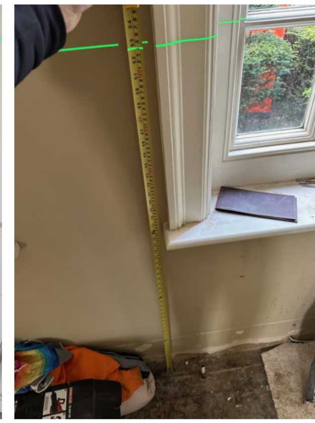
Picture 2 - Highest point of timber floor (1339mm = -50mm)
