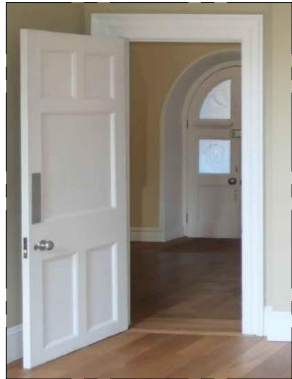
06 INTERNAL DOOR 02 - RETAIN EXISTING GROUND FLOOR- R03 FORMAL LIVING
