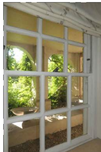
11 W. ARCHITRAVE 10 - RETAIN EXISTING LGF - R010 EN-SUITE 01
