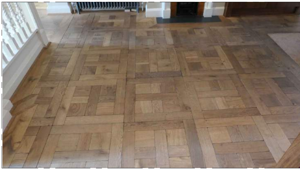
01 FLOORING 01 - RETAIN EXISTING GROUND FLOOR - R01 ENTRANCE HALL
