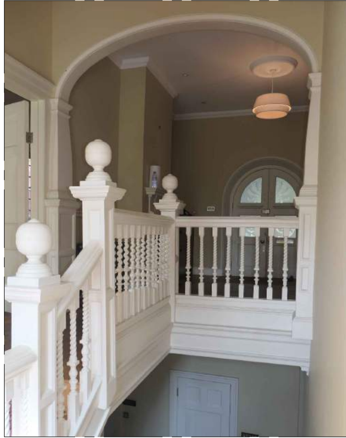
01 STAIRCASE 01 - RETAIN EXISTING PHOTOGRAPH 01
