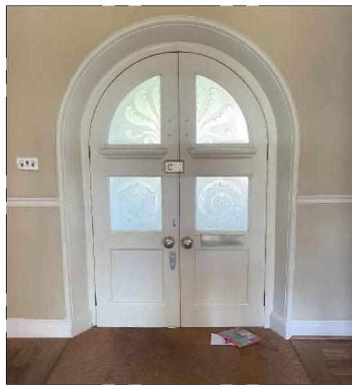
01 EXTERNAL DOOR 01 - RETAIN EXISTING GROUND FLOOR- R01 ENTRANCE HALL
