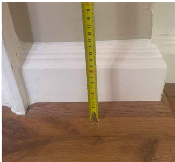
05 EXISTING SKIRTING 01 - RETAIN EXISTING GROUND FLOOR - R01 ENTRANCE FLOOR
