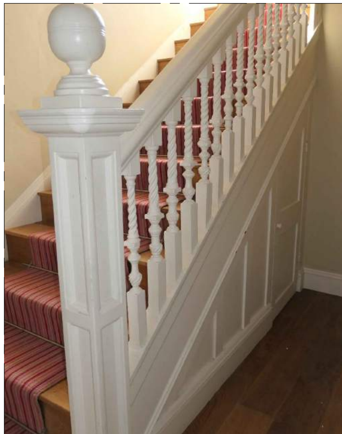
03 STAIRCASE 01 - RETAIN EXISTING PHOTOGRAPH 03
