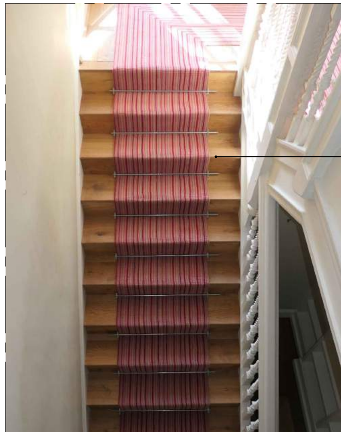
04 STAIRCASE 01 - RETAIN EXISTING PHOTOGRAPH 04
