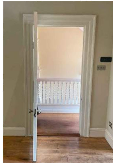
07 INTERNAL DOOR 03 - RETAIN EXISTING GROUND FLOOR- 04 KITCHEN
