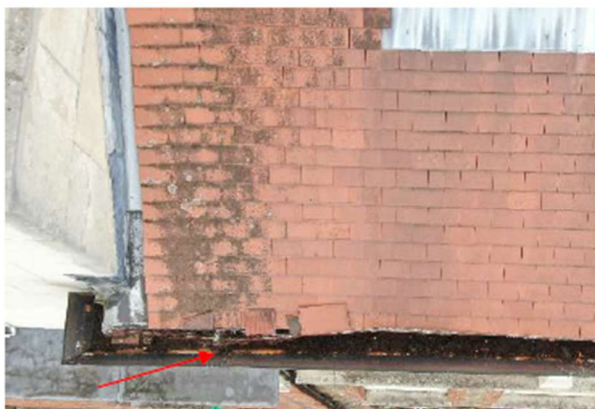
Figures 4 and 5: slipped tiles caught in snowguards and resting on parapets. Broken Defective Stone Copings. Playground directly below.
