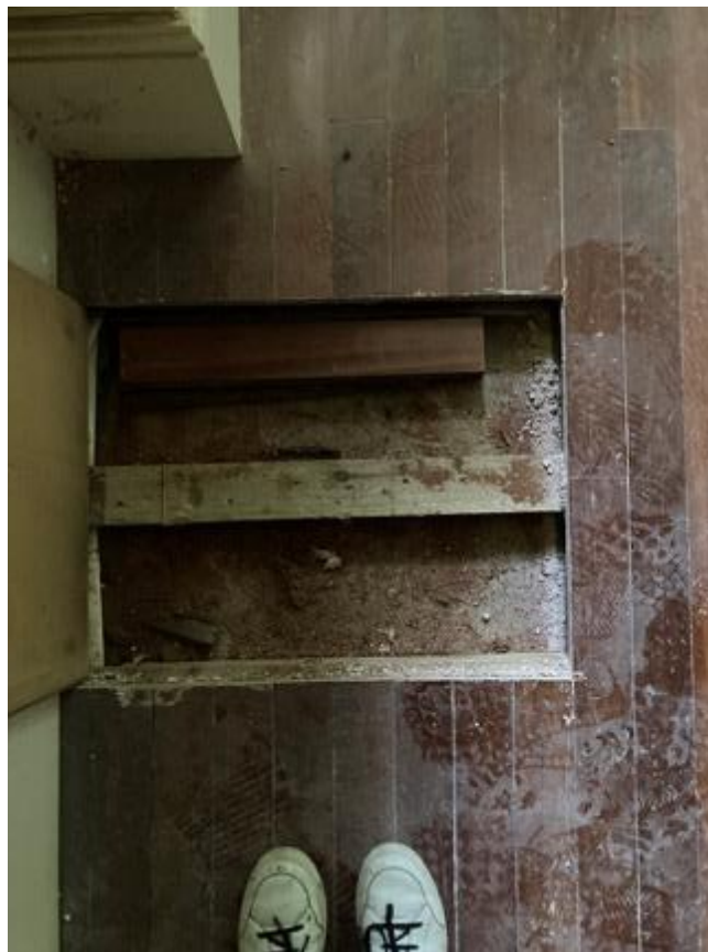
View of the replaced wooden floor and concrete base
