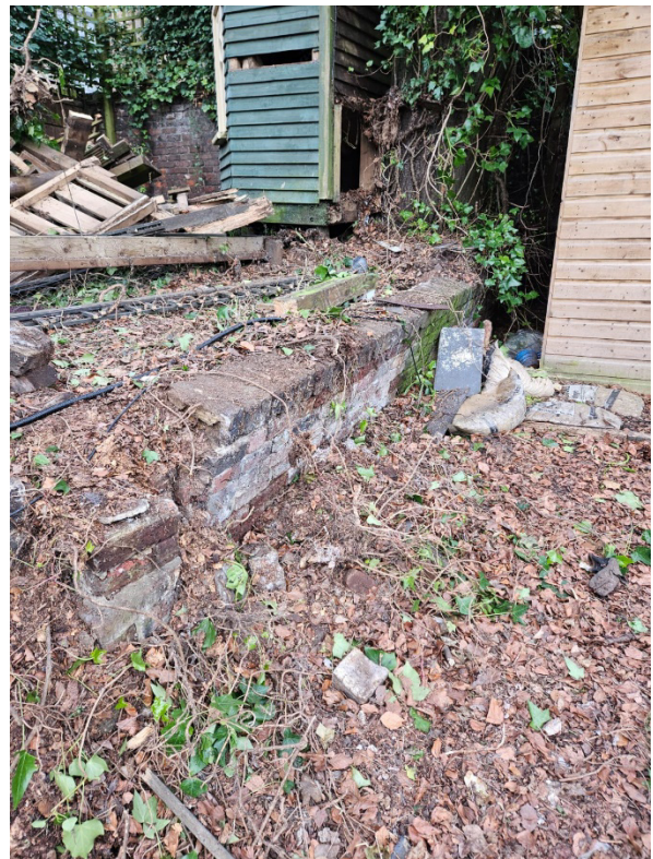
Wall when seen after removal of trellis and ivy, showing collapse and dangerous lean towards No. 9
