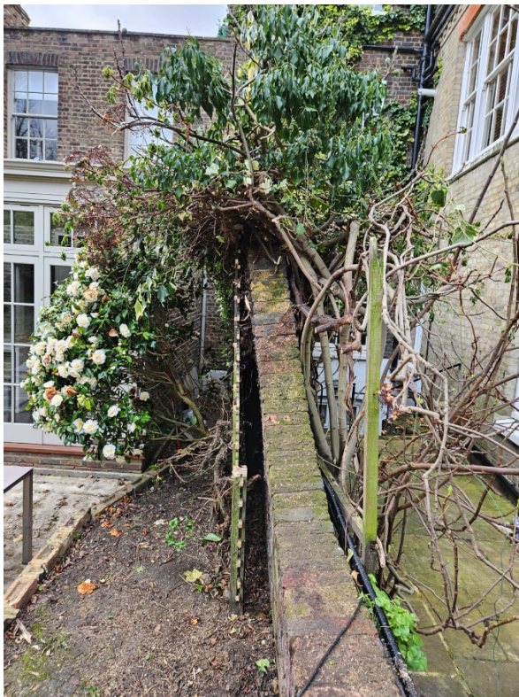
Wall when seen after removal of trellis and ivy, showing collapse and dangerous lean towards No. 9
