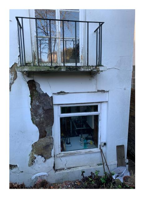
At ground floor the original configuration of the rear parlour room double hung sash windows is to be reinstated - eliminating the existing double doors and fanlights. The balcony railings are also to be replaced to an appropriate original pattern.
