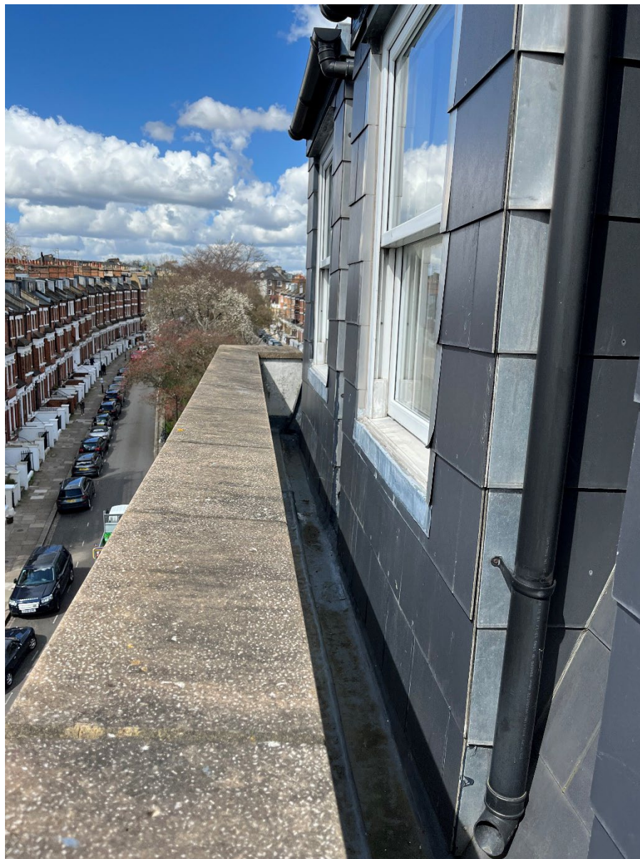
Photo 3 – existing box gutter uPVC window, new units to match. Newly formed opening to be finished at low level with a weather proofed external insulated wall finished externally in slates to match.
