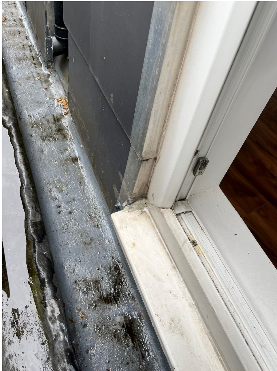
Photo 5 – threshold of existing door openings too low, causing damp ingress problems.
