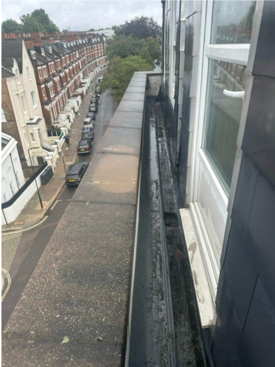
Photo 1 – roof level box gutter, showing existing upvc door, to be stripped out and replaced with a upvc window to match the existing window units on the elevation.
