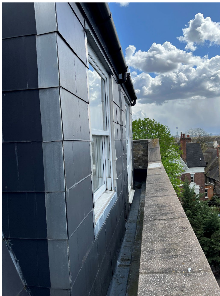
Photo 2 – existing box gutter uPVC window, new units to match. Newly formed opening to be finished at low level with a weather proofed external insulated wall finished externally in slates to match.
