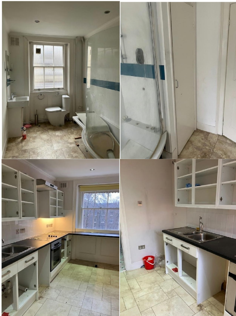
Figure 2 - Photos showing the current status of Rm 306 and Rm 308
