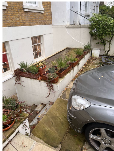
View of concrete store cupboards to front well
