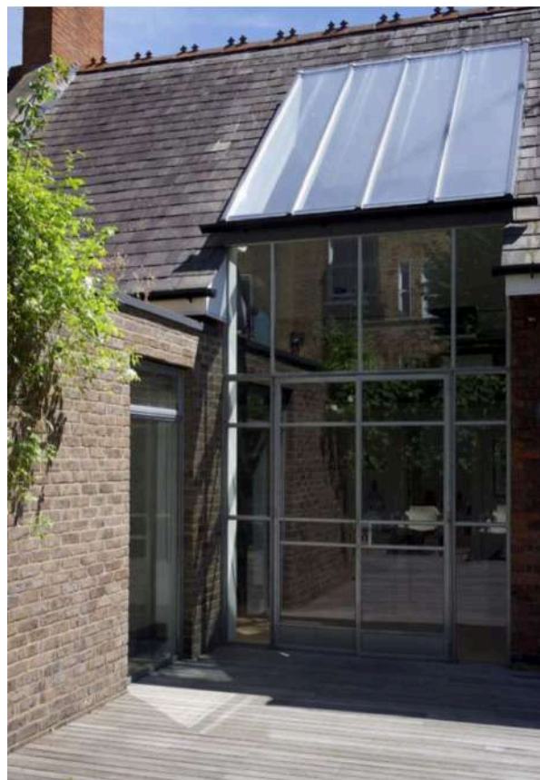
Image: Photograph showing the galvanised steel Crittall windows and doors installed at 4 Primrose Hill Studios
