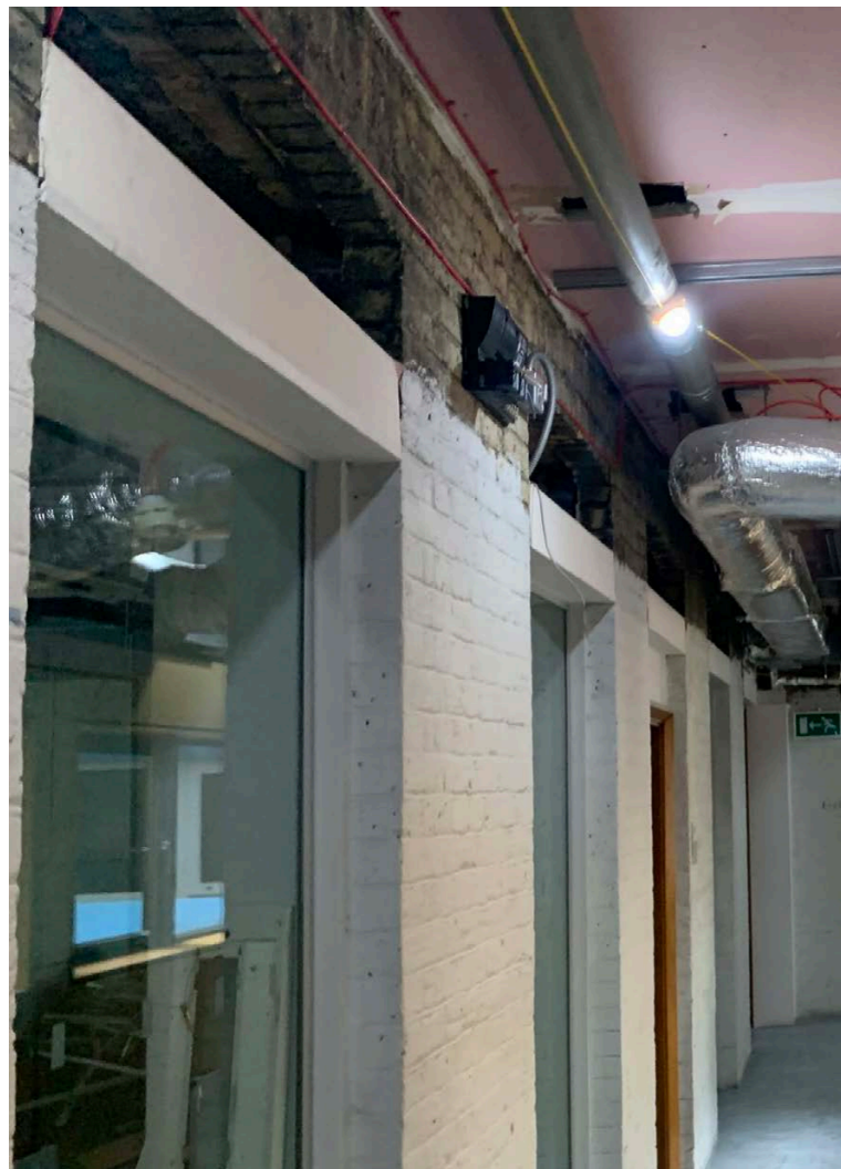
North corridor with exposed brickwork and arches from former external wall
