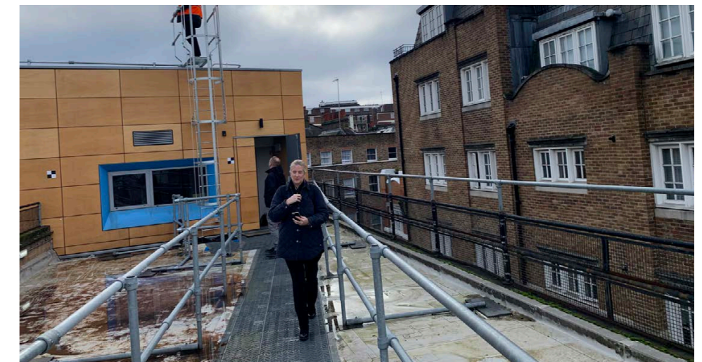
15. Lower roof looking south
