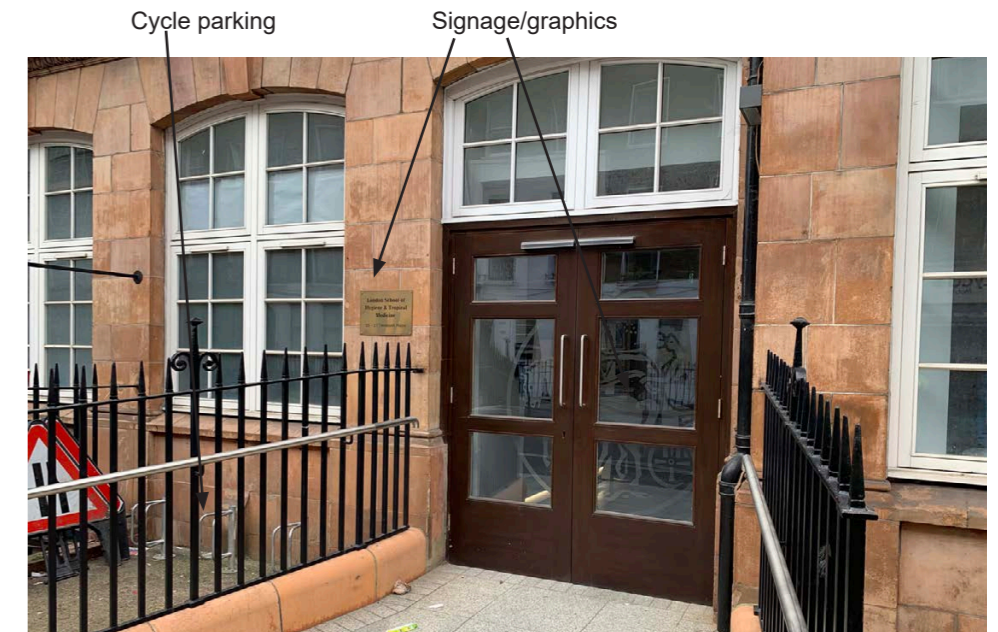
8. TP1 eastern end current (temporary) main entrance
