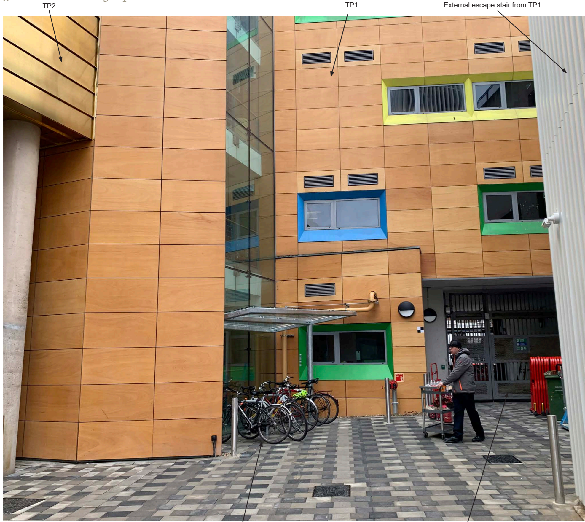
10. Courtyard looking south
