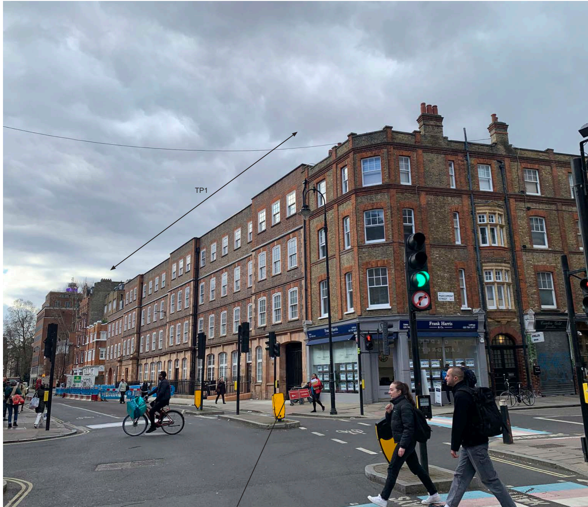
7. TP1 looking west
