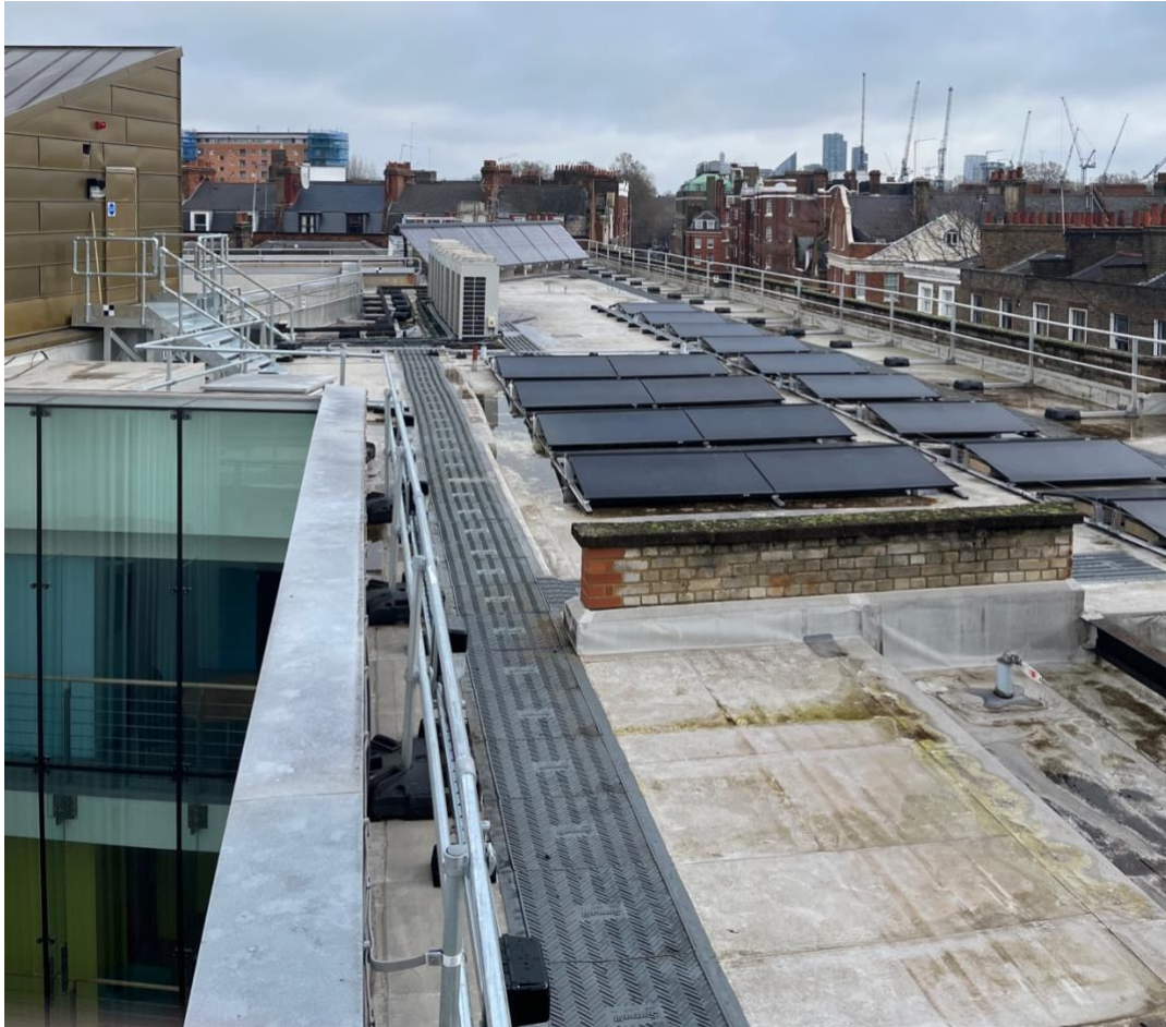
Existing flat roof with building services plant and PV units
