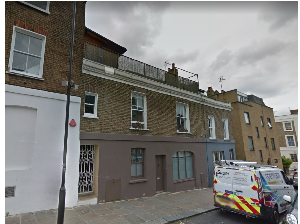
○ Street view of 10 York Rise
