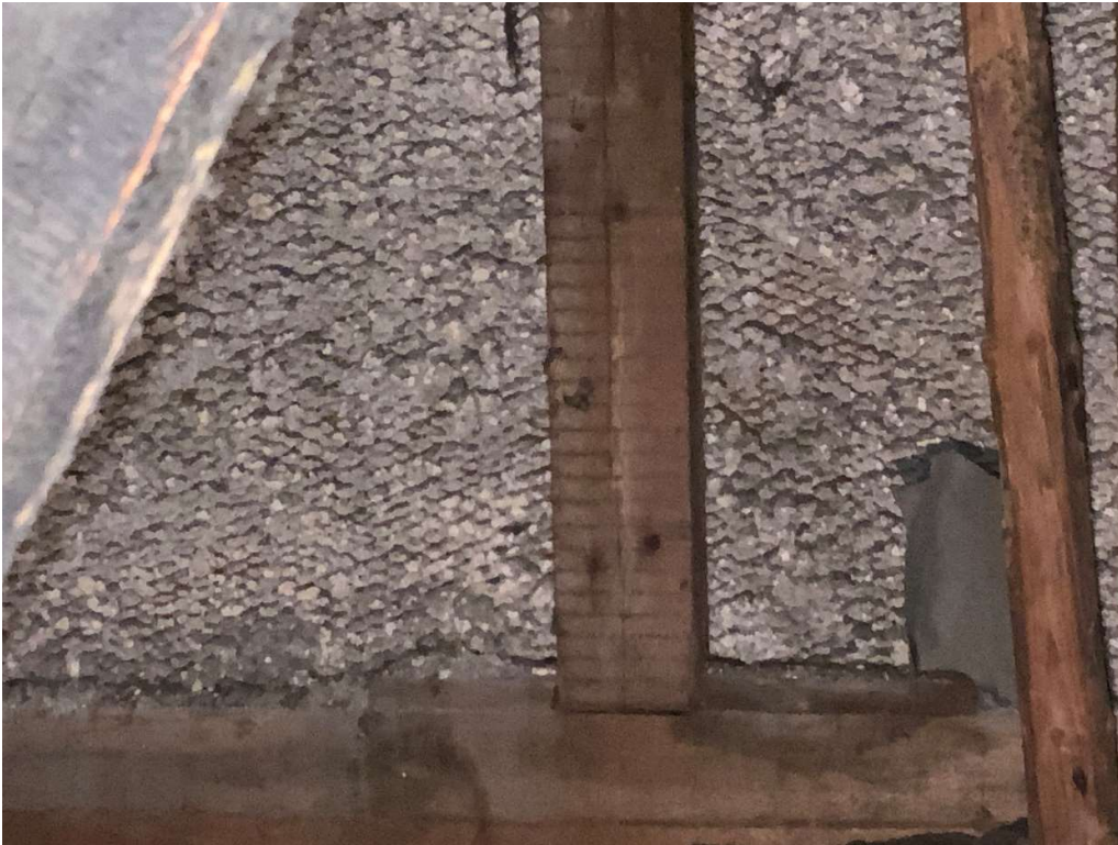
South gable with modern sawn timbers with render on modern metal lath
