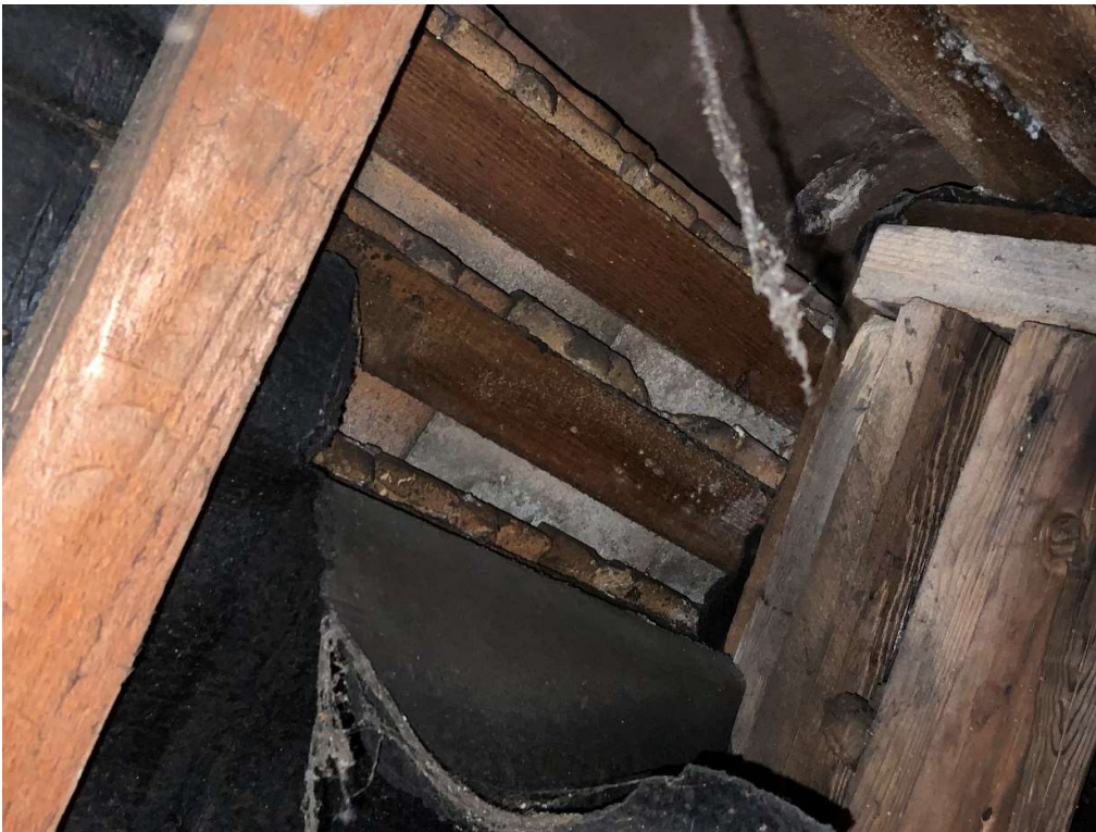
Modern rafters and bituminous felt with modern battens over supporting modern concrete tiles
