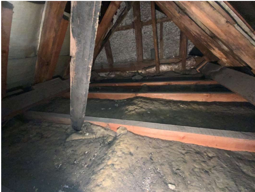
Modern rafters with saw marks and ceiling joists with render on modern metal lath to south gable
