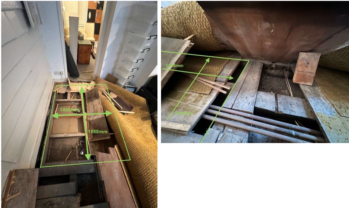
Marked-up-up image showing the location of the original stairwell which has been infilled with modern timber joists. These are to be removed and the stairwell reinstated to its original configuration, retaining all historic fabric unaltered.
