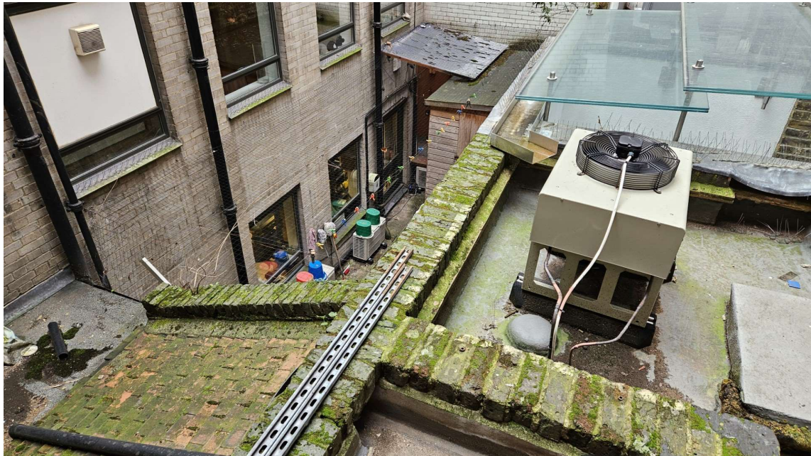
VIEW LOOKING SOUTH TO COURTYARD AND TOWARDS NO. 2/3 SCALA STREET
