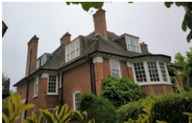
Photo 3, 21.05.2024: Front and left side
