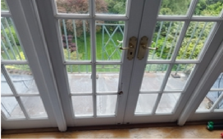
Photo 13, 21.05.2025: French door from inside, garden view
