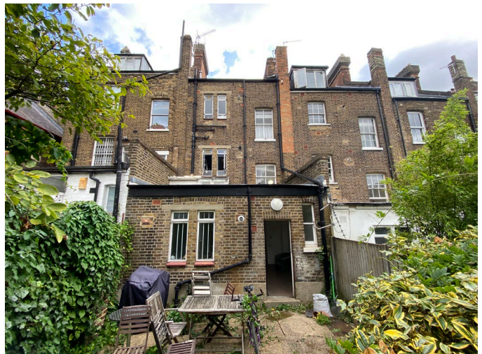
Rear elevation (site survey photo 22.08.23)
