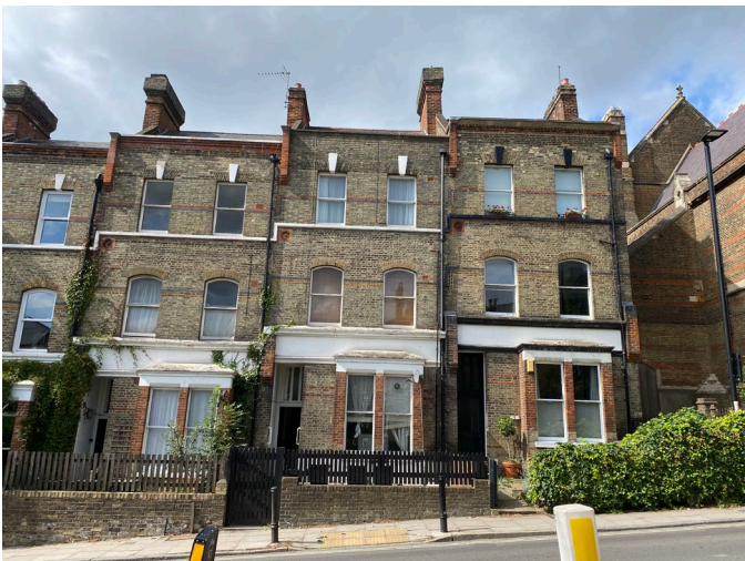
Front elevation (site survey photo 22.08.23)
