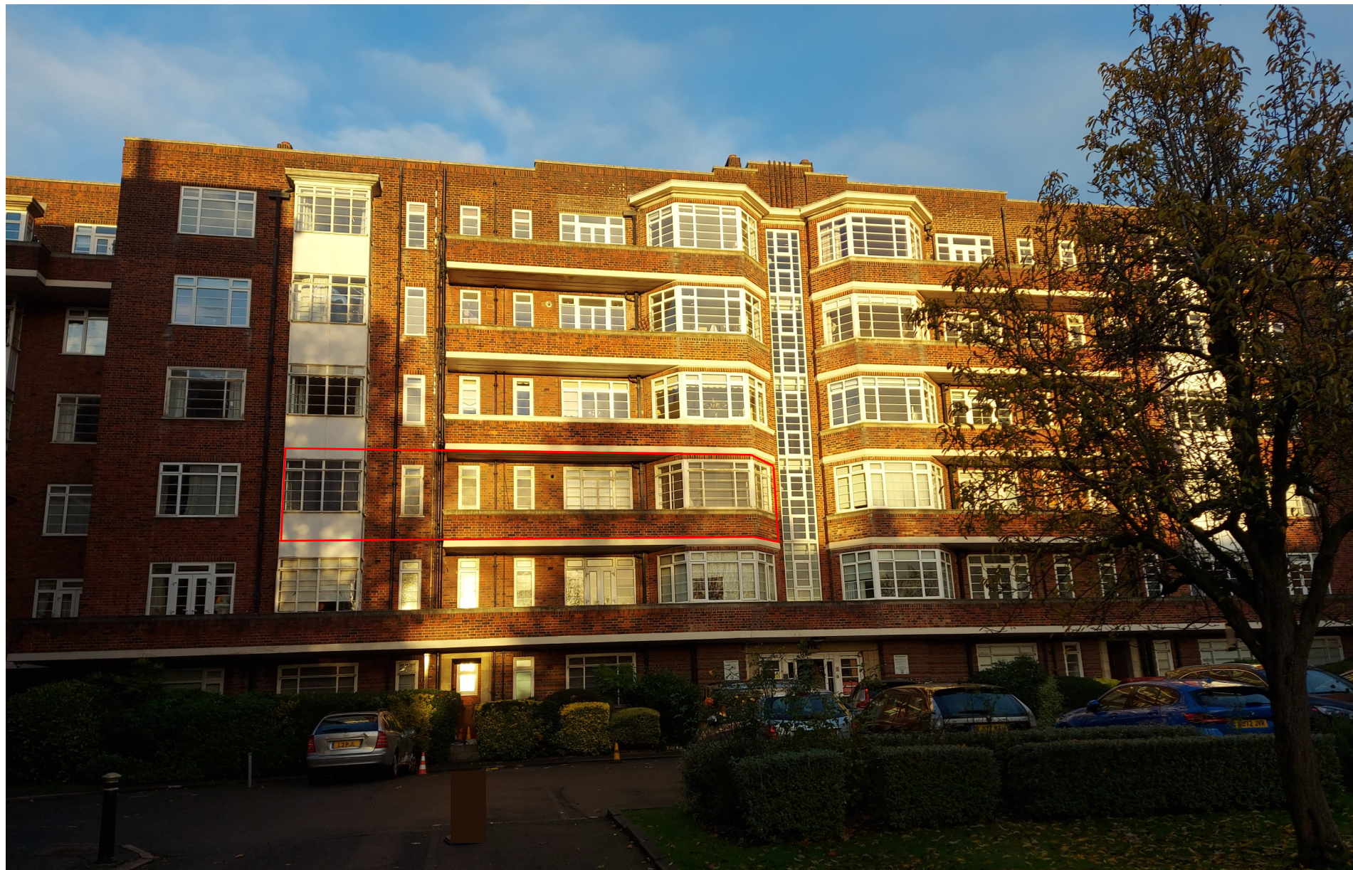
FLAT 57 second floor (outlined in red) HILLFIELD COURT BELSIZE AVENUE, LONDON NW3 4BG Ref: 597 PHOTO-1
