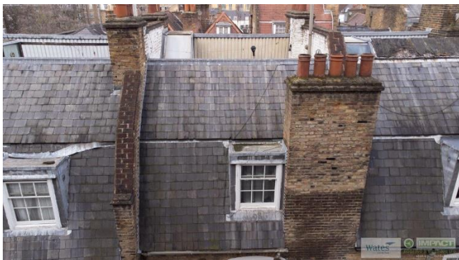
Photo 1: Pitched Roof Coverings 14 Dombey Street (Rear)
