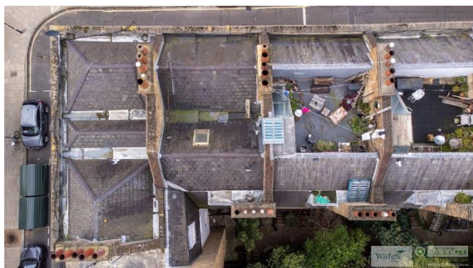
Photo 11: Aerial View including 10 and 11 Dombey Street
