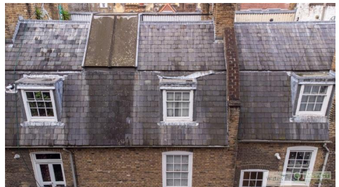
Photo 2: Pitched Roof Coverings 13 Dombey Street (Rear)
