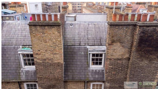
Photo 5: Pitched Roof Coverings 10, 11 Dombey Street (Rear)
