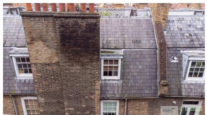
Photo 4: Pitched Roof Coverings 11, 12, 13 Dombey Street (Rear)
