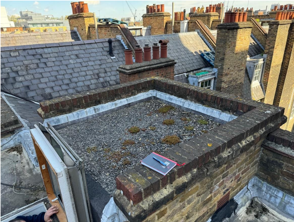
Figure 2: Picture showing existing lift overrun
