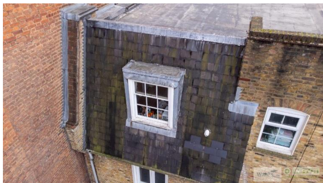
Photo 9: Bevan John House (Rear)
