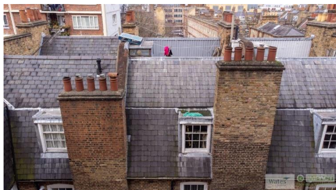
Photo 6: Pitched Roof Coverings 9, 10 Dombey Street (Rear)
