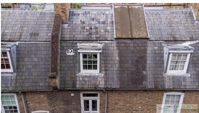
Photo 3: Pitched Roof Coverings 13 Dombey Street (Rear)
