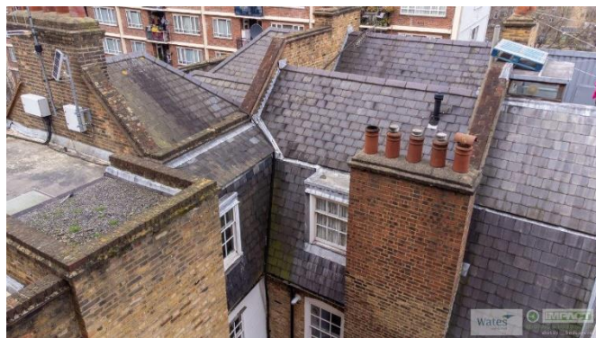
Photo 10: Bevan John House Lift Shaft (Rear)
