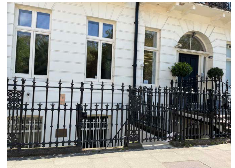
Existing Gate for Previous Platform Lift and Call Point
