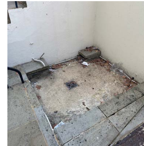
Existing Lift Pit
