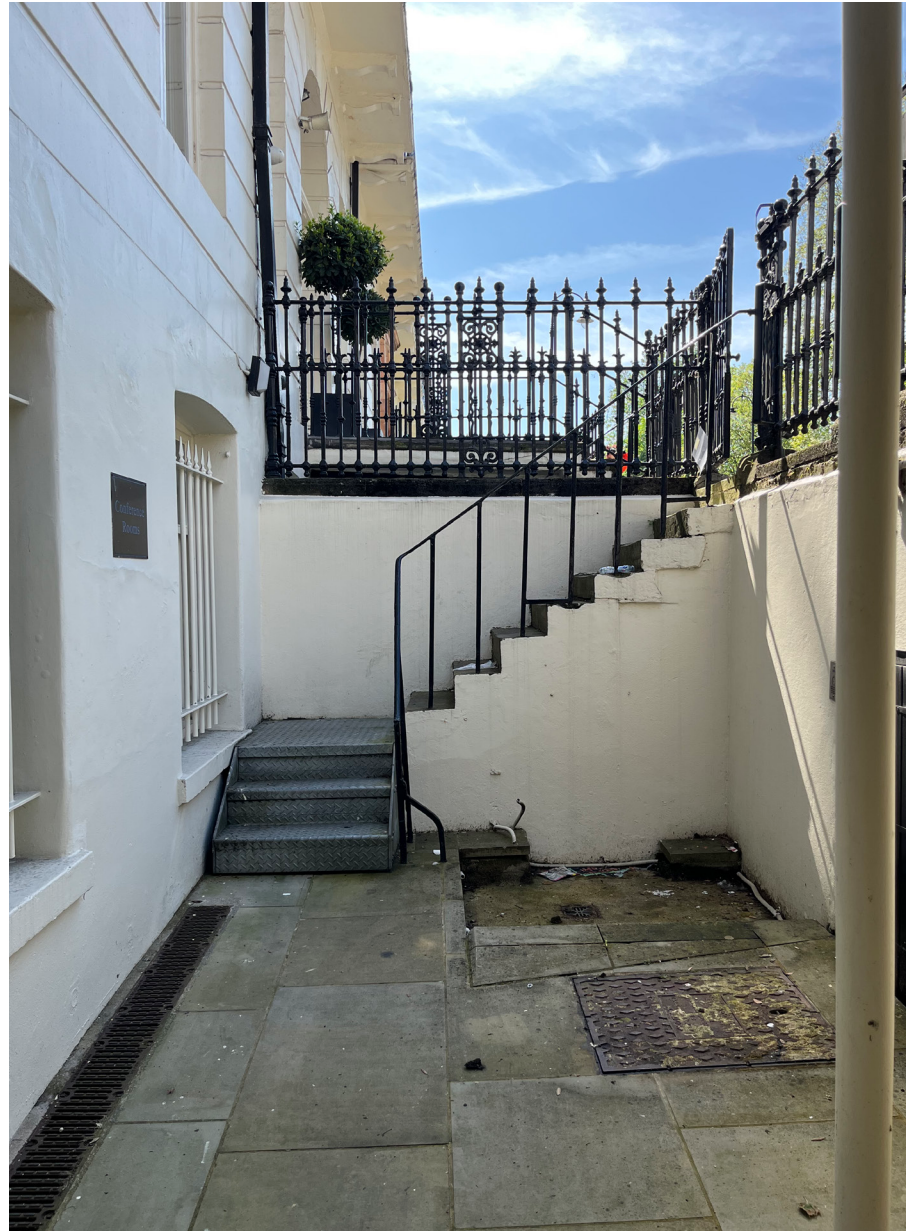
Existing Lightwell at No. 57
