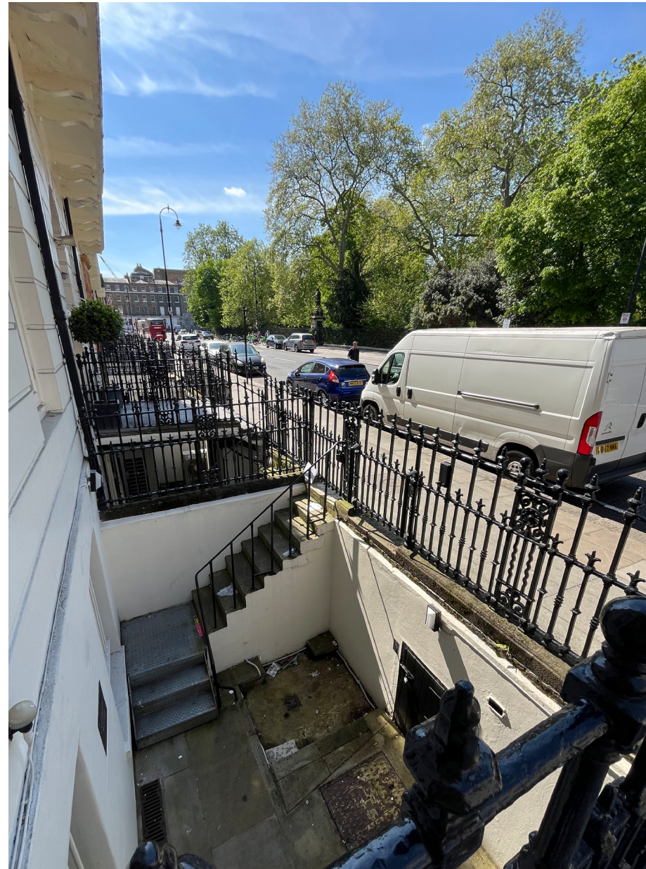
Railings and Gates at Pavement Level
