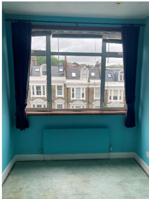
12. Site visit photograph, one side of existing front dormer.
