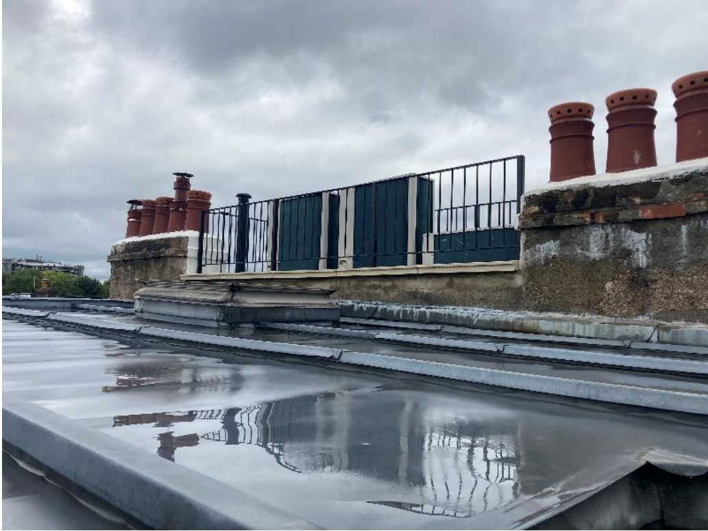
15. Site visit photograph, existing roof and neighbouring plant arrangement.
