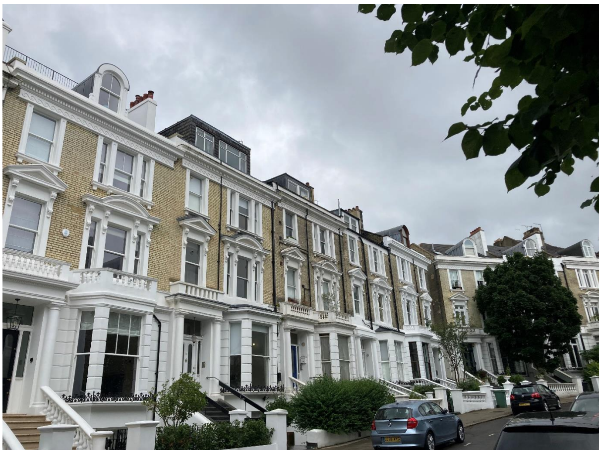
6. Site visit photograph, street scene. Host site with large existing front dormer.
