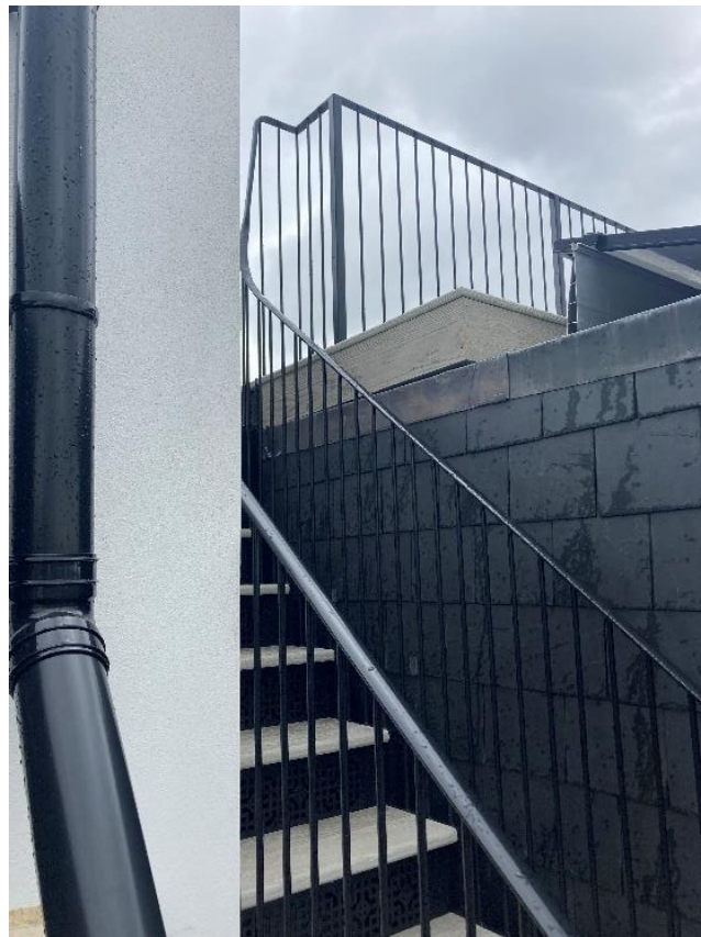
16. Site visit photograph, existing neighbouring access to roof.
