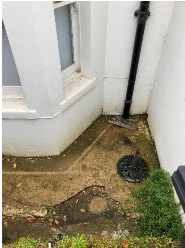
8. Site visit photograph, Front light well.
