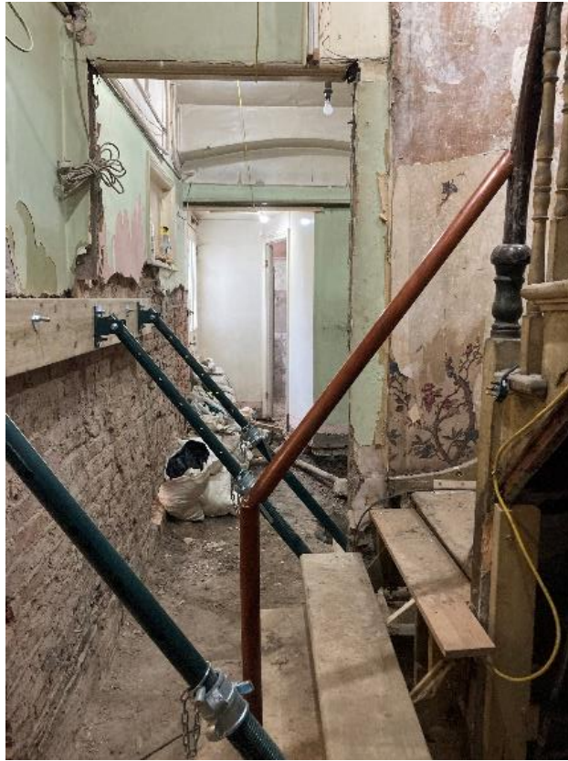
9. Site visit photograph, existing condition at lower ground floor.
