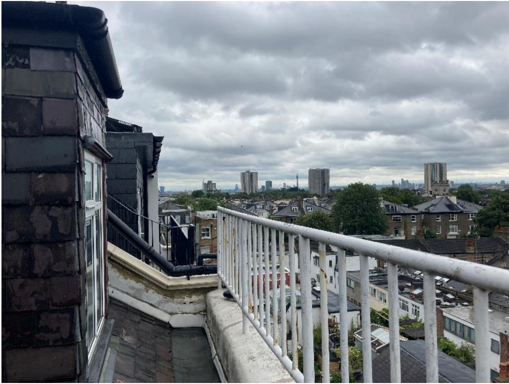
13. Site visit photograph, existing rear balcony railing.
