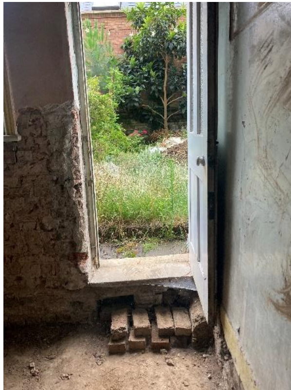
10. Site visit photograph, lower ground floor view to rear.
