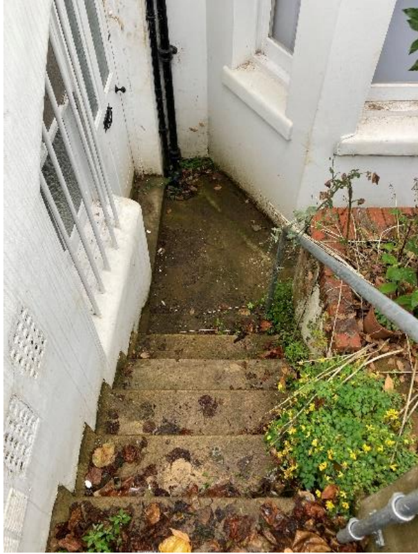
7. Site visit photograph, front light-well.
