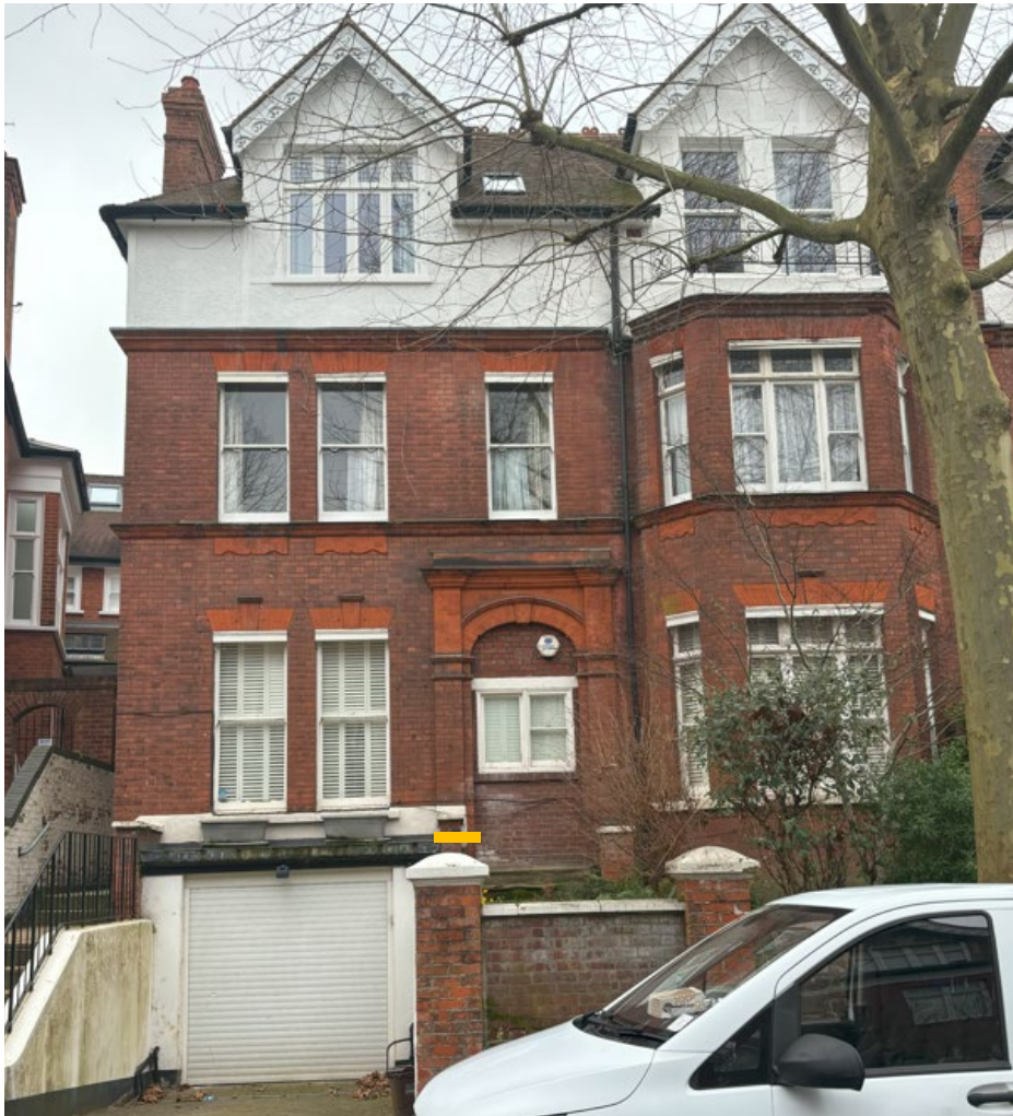
Figure 1 Front façade view
