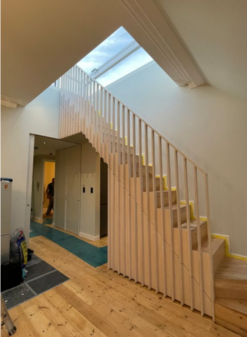
Figure 8 Roof terrace access stairs from second floor Flat C living room.
