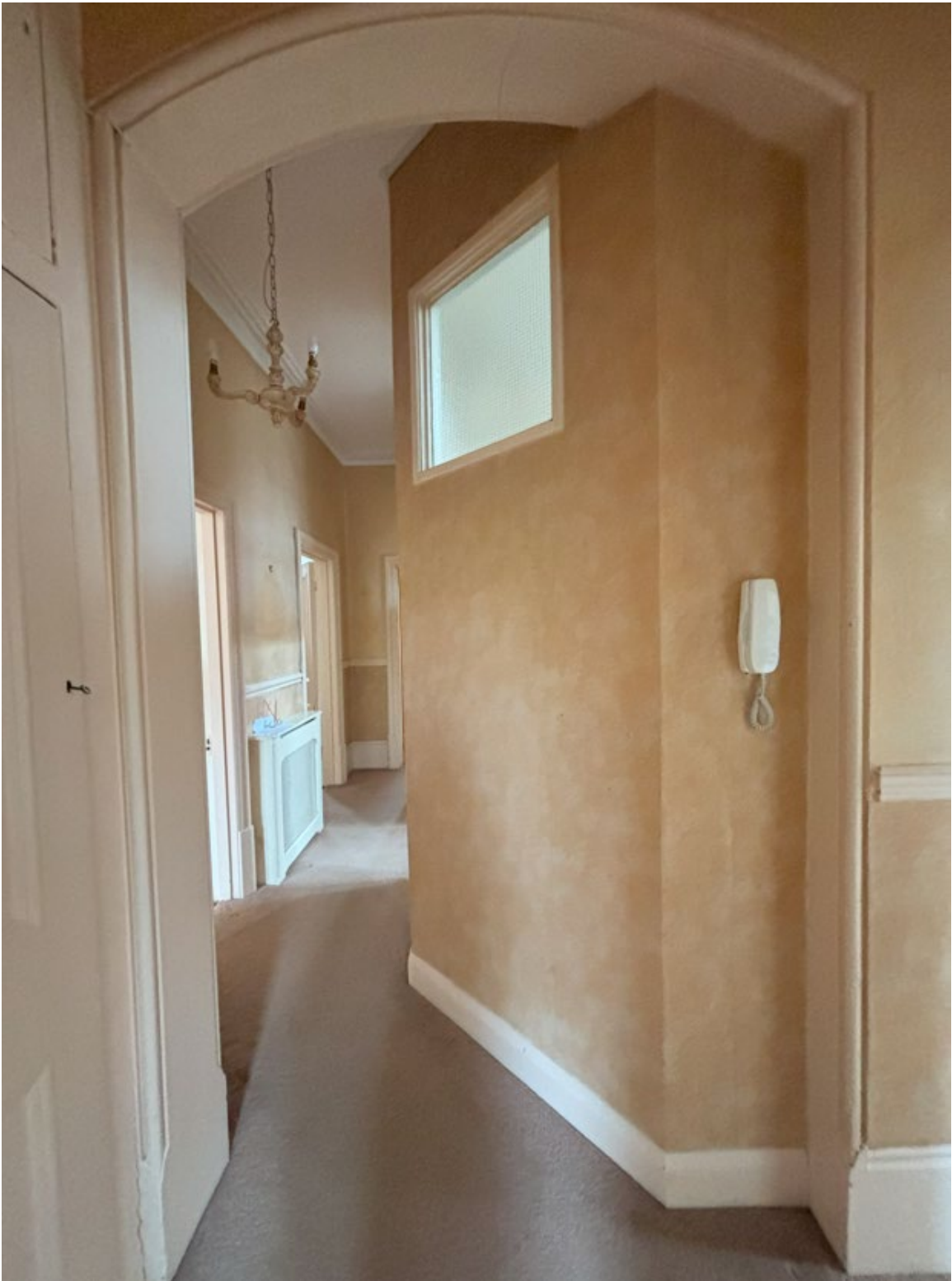
Figure 6 1970s partitioning to close off first floor Flat B from stairwell
