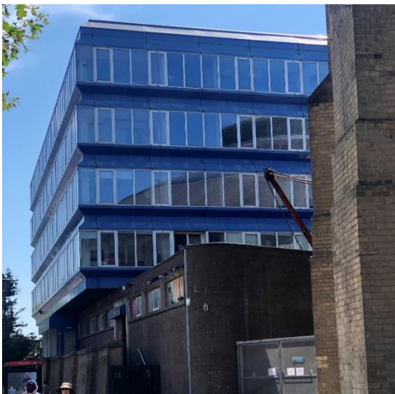
Office Building and Dressing rooms
