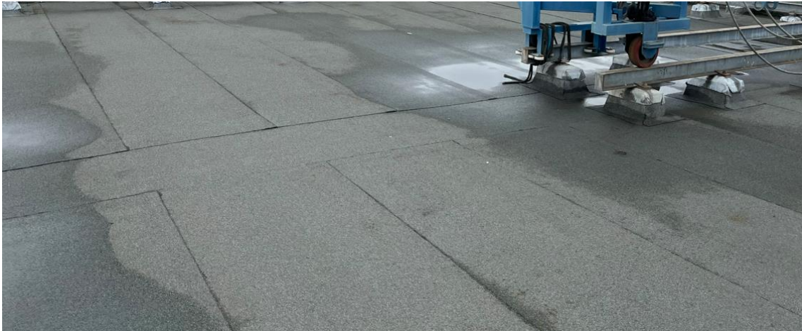
Figure 22 Roofing felt – office
