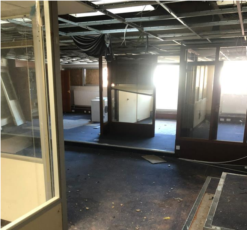
Figure 20 Internal glazed partitions
