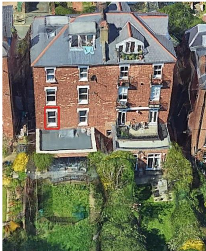
Figure 1 – The rear elevation of the existing building with the window that has been replaced outlined in red.
