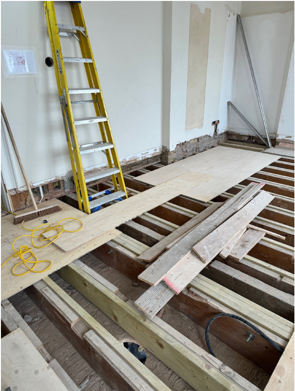
Image of existing, strengthened joists
