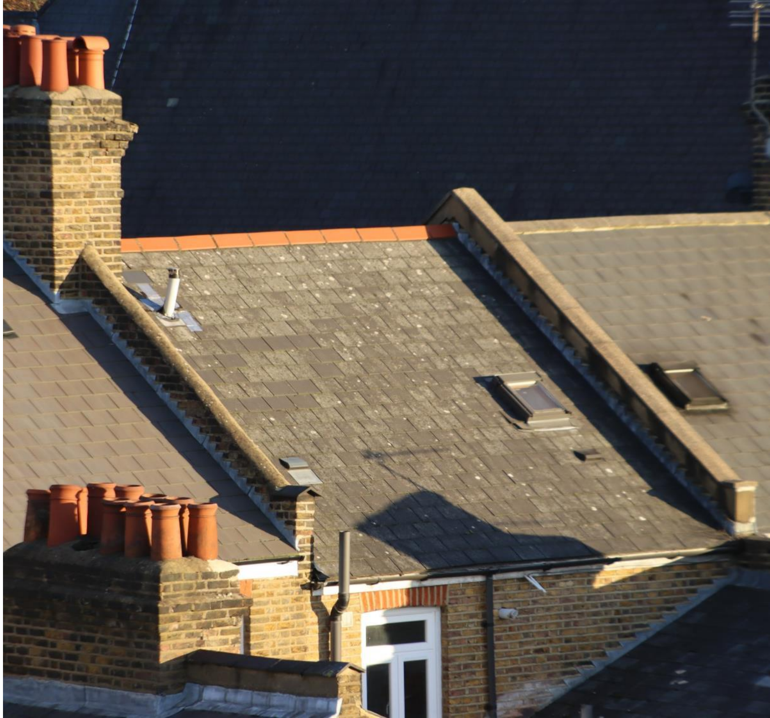
Roof Rear slope
