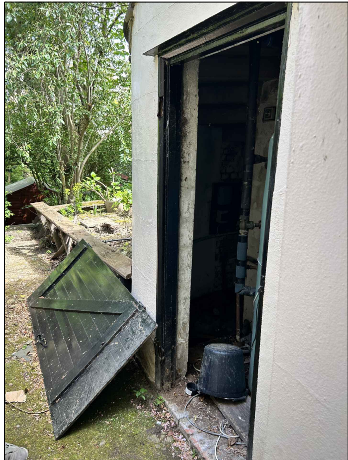
Existing Ledged & Braced Door
