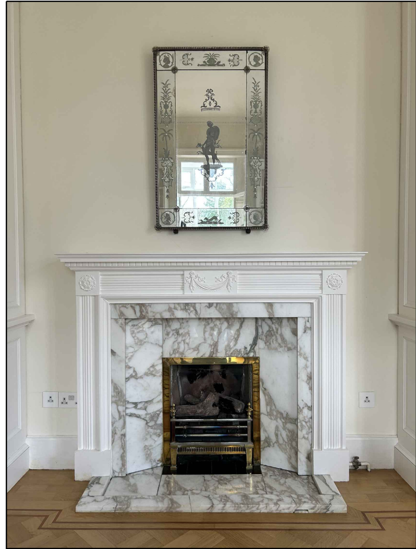
Existing RG05 Fireplace
