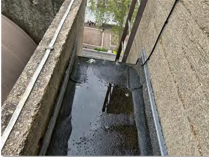
IMG_3887 (Area 3) Service Shaft Connection between service shafts
