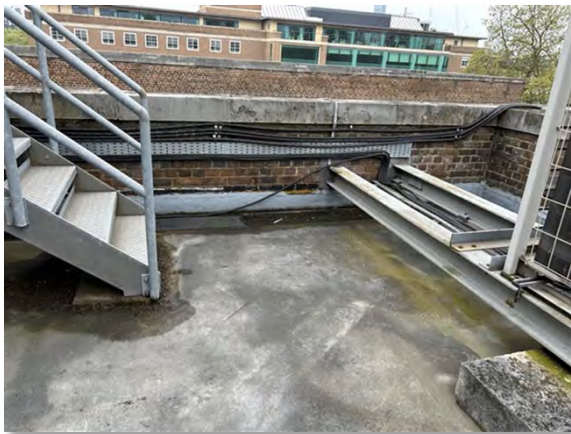
IMG_3834 (Area 9) Plant support steels pocketed into brick upstand
