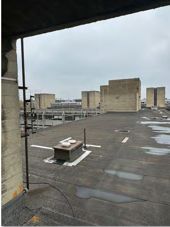
IMG_2740 (Area 2) Main Roof Redundant ventilation housing to be removed
