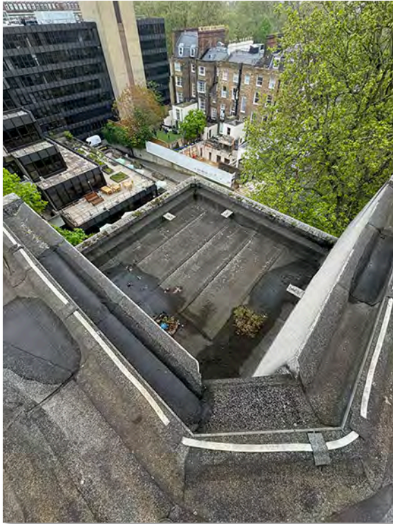
IMG_2747 (Area 5) Showing redundant anchor blocks to perimeter upstand & wall, to be removed. Also showing formed gutter to roof Area 2
