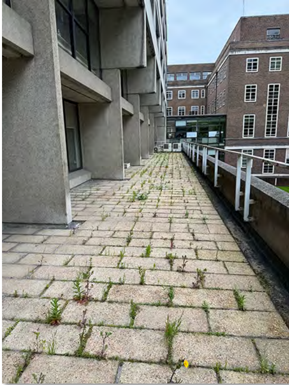
IMG_2894 (Area 7) Concrete paving over bituminous membrane system
