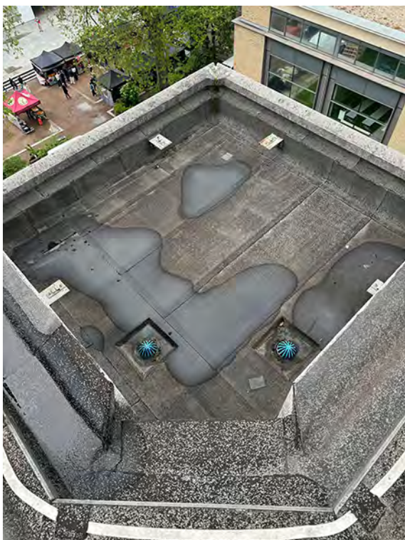
IMG_2747 (Area 5) Showing redundant anchor blocks to perimeter upstand & wall, to be removed. Also showing formed gutter to roof Area 2
