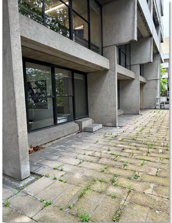
IMG_2888 (Area 7A) Stepped access onto terrace
