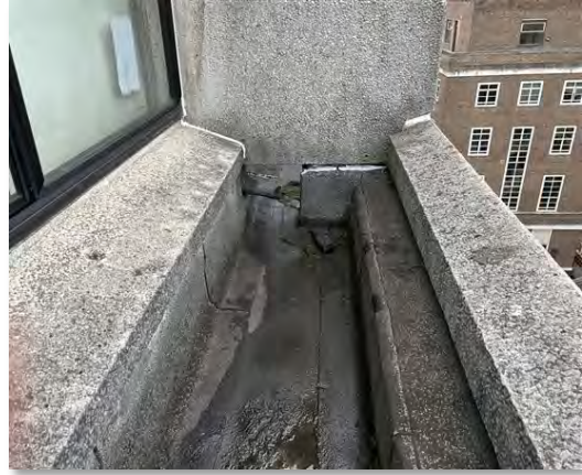
IMG_3923 (Area 4) Gutter
