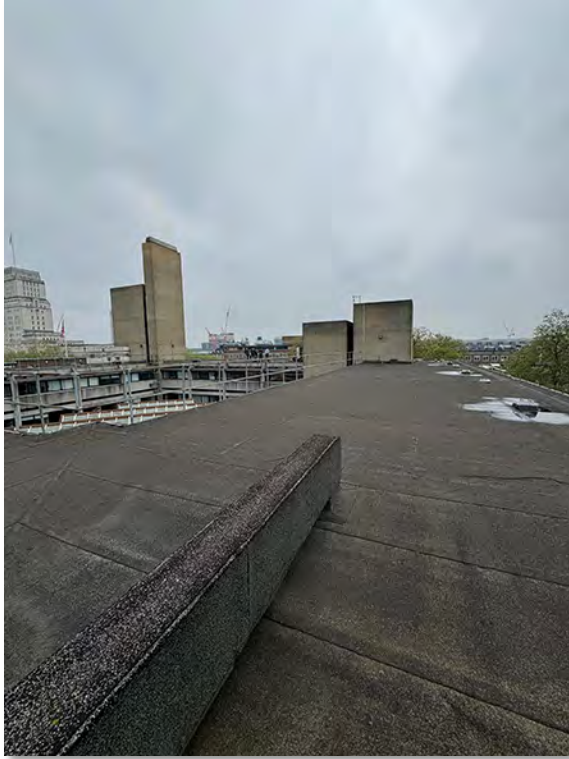
IMG_2754 (Area 2) Main Roof
