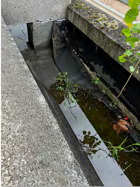
IMG_2926 (Area 4) Gutter
