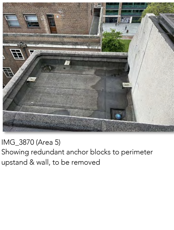
IMG_2753 (Area 5) Showing redundant anchor blocks to perimeter upstand & wall, to be removed. Also showing formed gutter to roof Area 2
