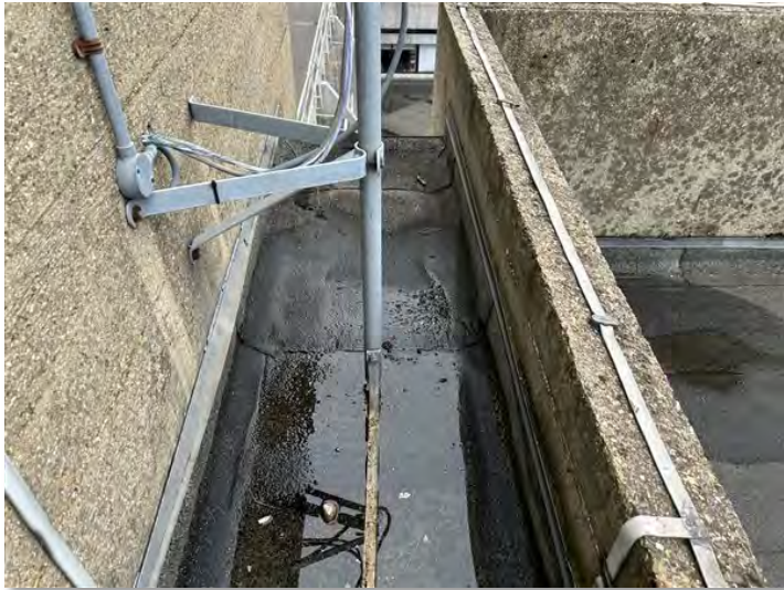
IMG_3888 (Area 3) Service Shaft Connection between service shafts
