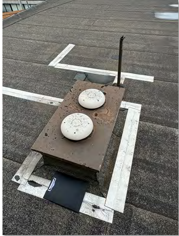
IMG_2742 (Area 2) Main Roof Redundant ventilation housing proposed to be removed
