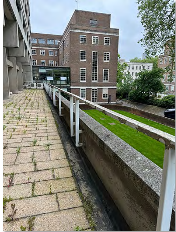
IMG_2897 (Area 7) Tubular steel balustrade to external perimeter of terrace
