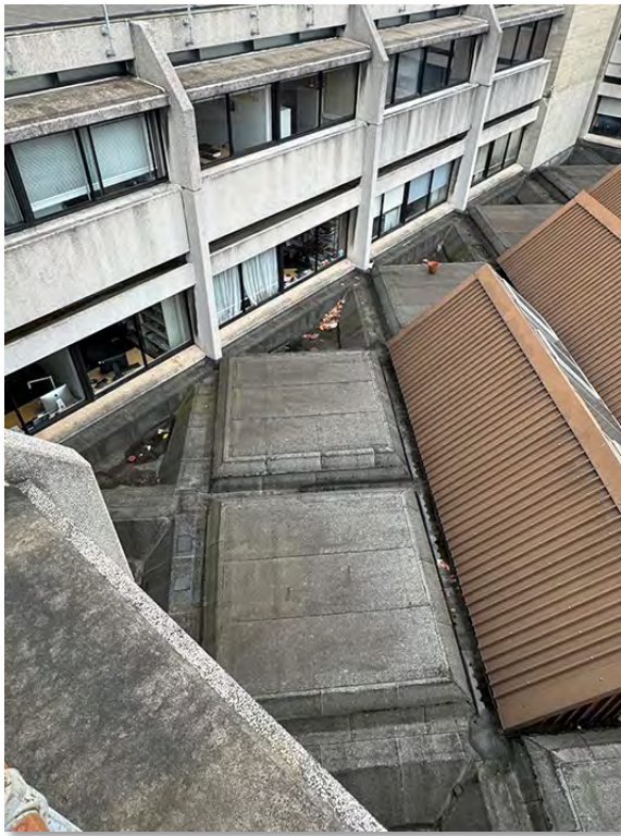
IMG_2744 (Area 1C) Library Roof Showing raised 'pedestal' sections of roof
