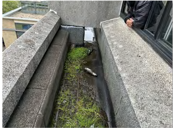
IMG_3916 (Area 4) Gutter
