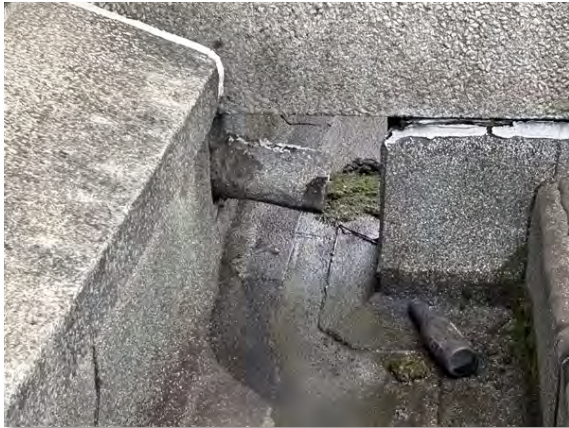
IMG_3924 (Area 4) Gutter
