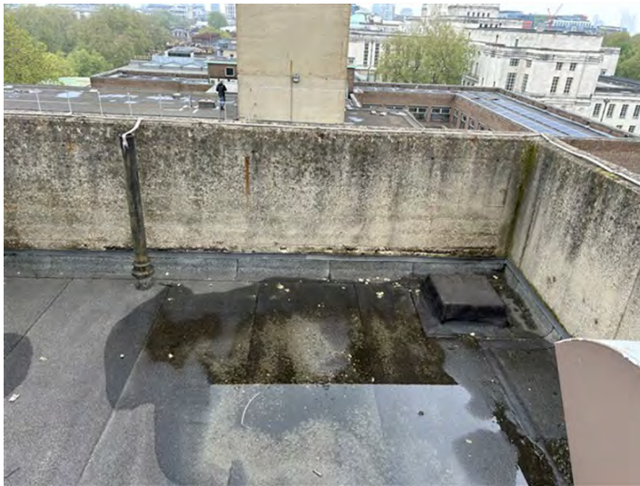
IMG_3885 (Area 3) Service Shaft Corner of service shaft roof
