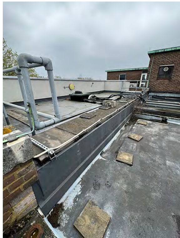
IMG_2719 (Area 9) Single ply membrane to upstand between roof Area 9 & 15
