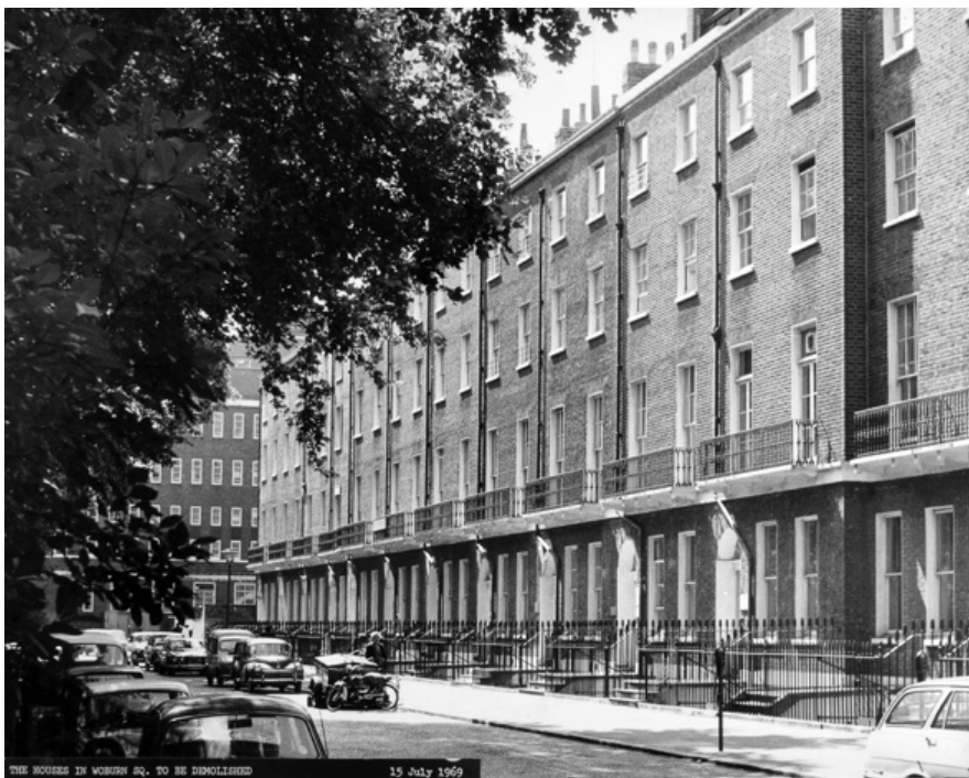
Woburn Square pre demolition 1969
