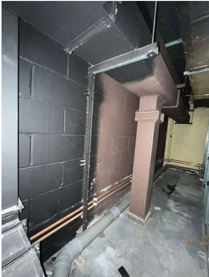
The above photograph shows the space to the rear of Unit 3 at UGF level. The MEP equipment will be modified to allow for access to the new proposed access door to be created in the block wall through to the south atrium.
