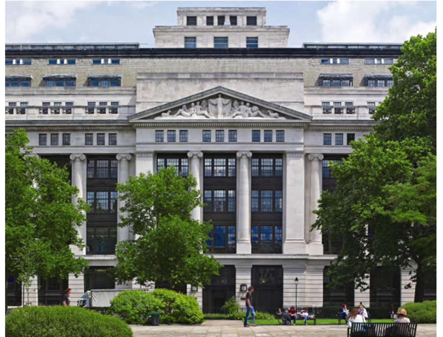
View from Bloomsbury Square towards building entrance
