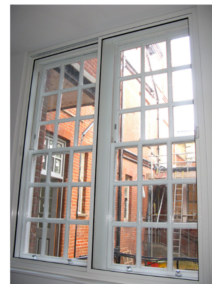
Selectagaze secondary glazing - Typical Installation
