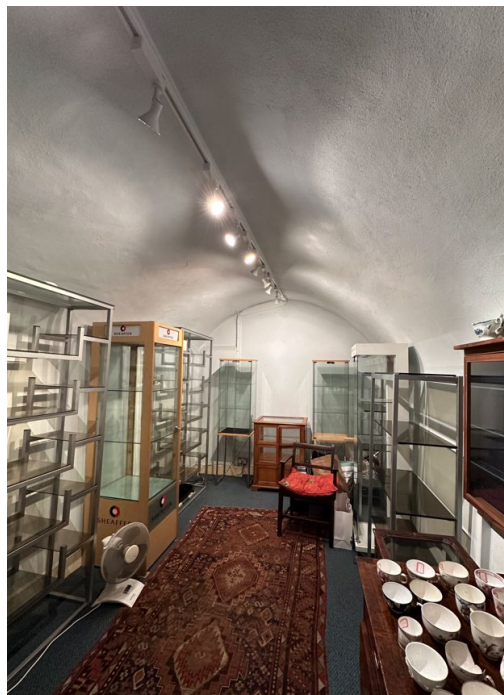
Figure 3: cementitious tanking of cellar 1
