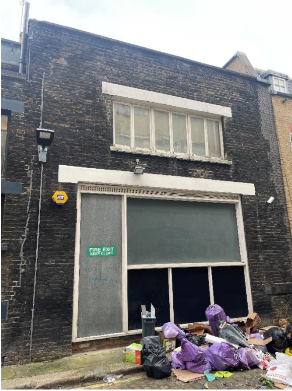
Above: Rear elevation from Percy Mews
