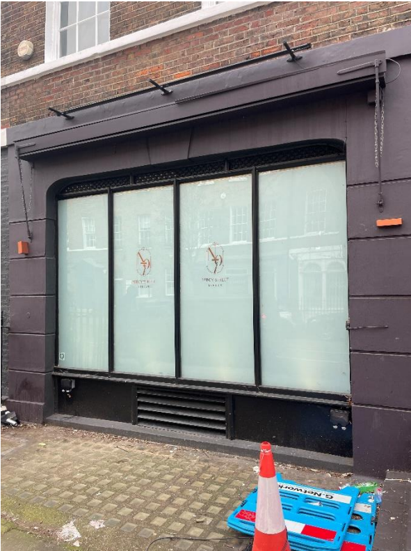
Above: Existing film treatment to front glazing (to be removed)
