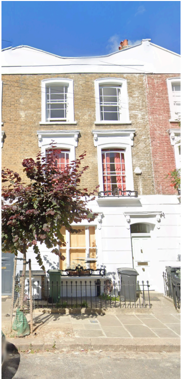
1.1 Existing front elevation on no.10 Healey Street
